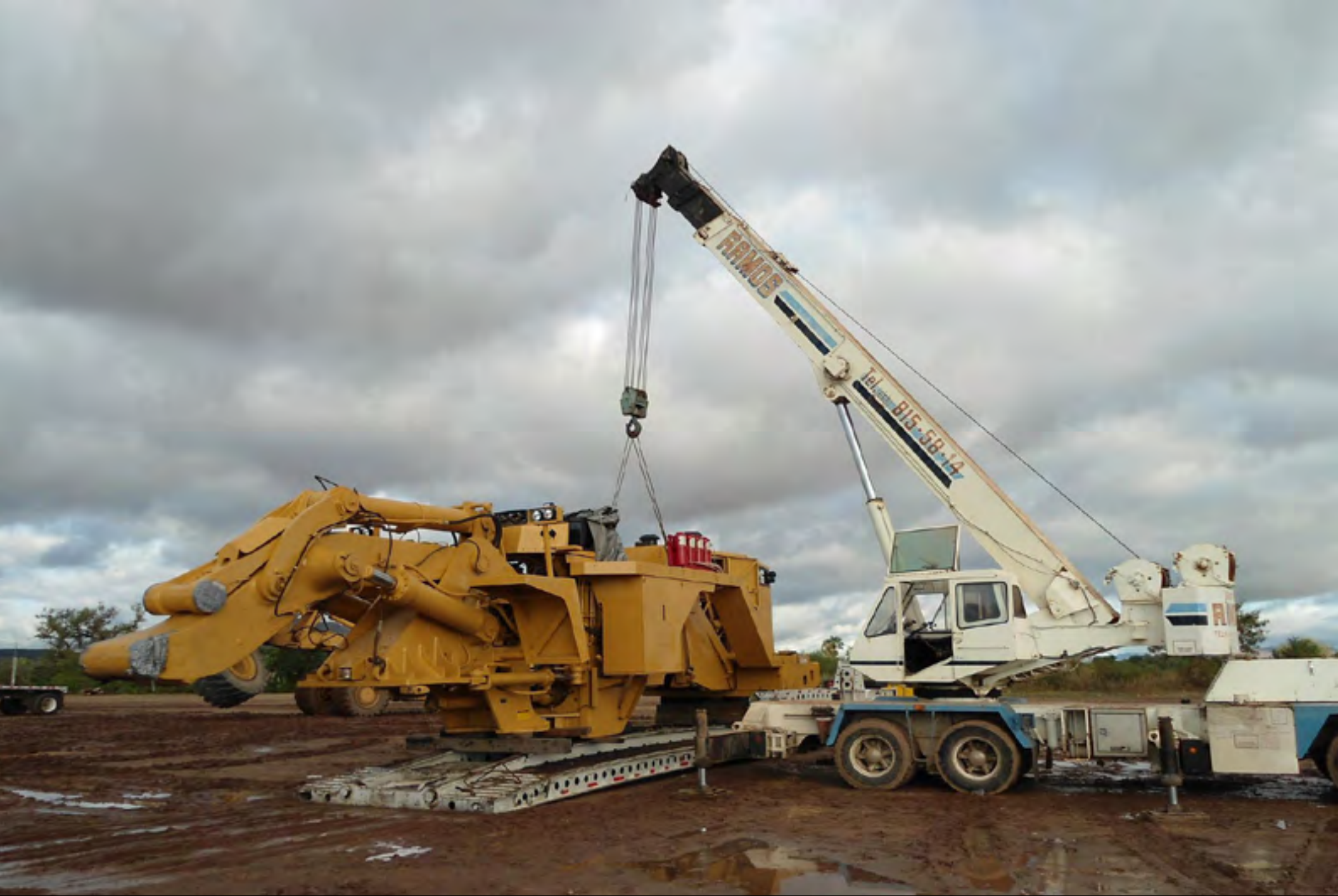
Assembly of front-end loader.
