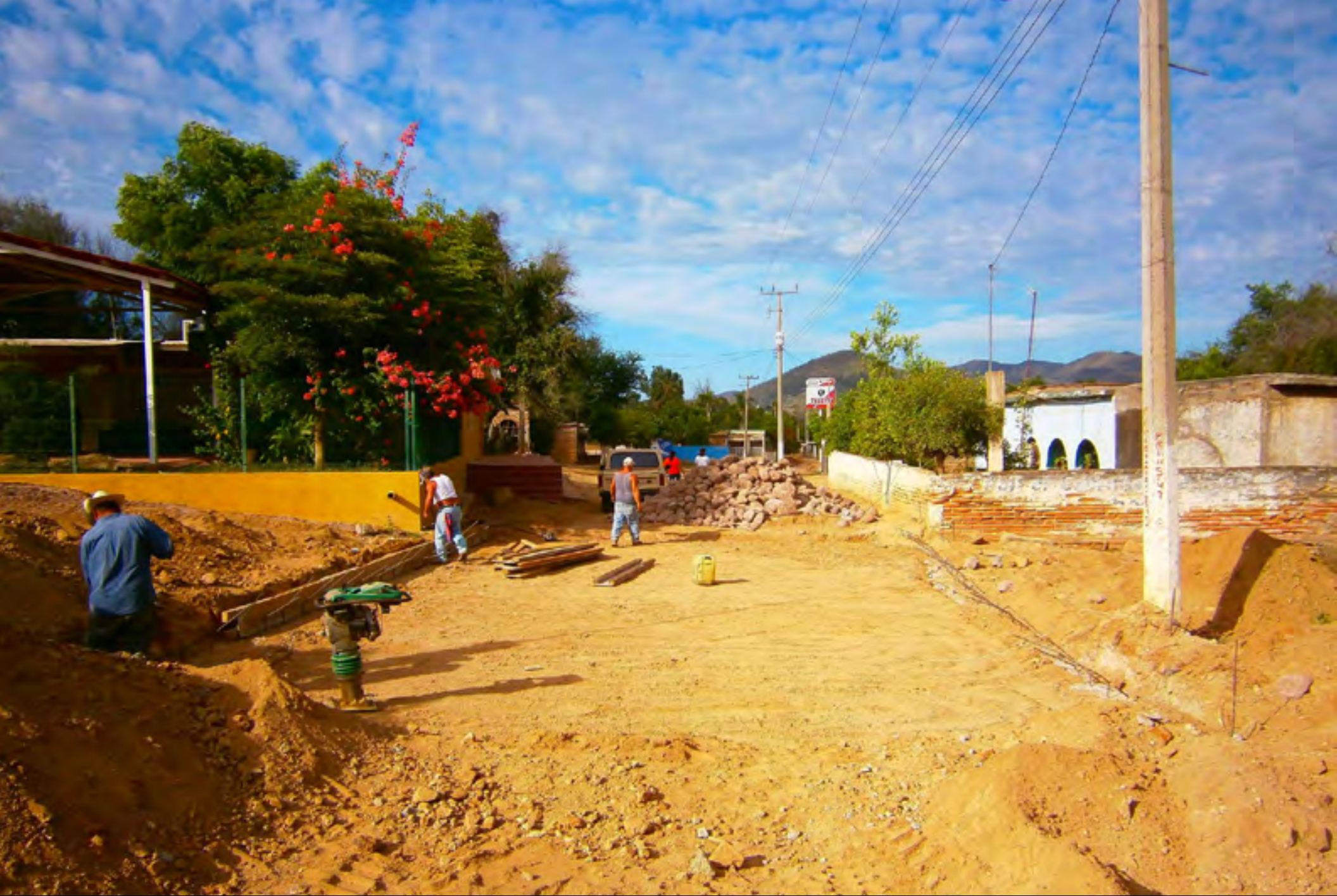
Upgrading the haul road between the Palmarito and El Gallo deposits.
