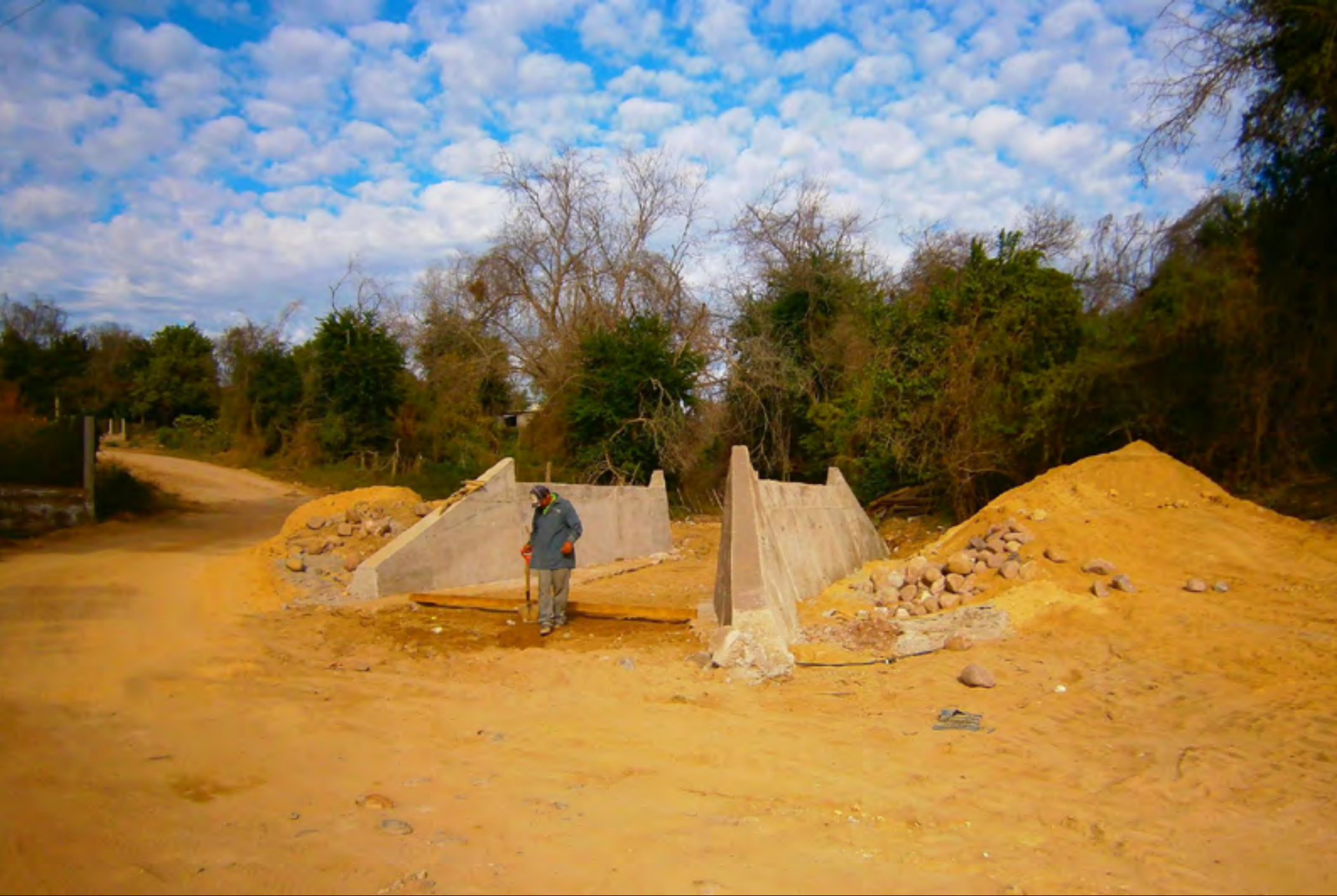
Bridge foundation for the haul road between Palmarito and El Gallo.
