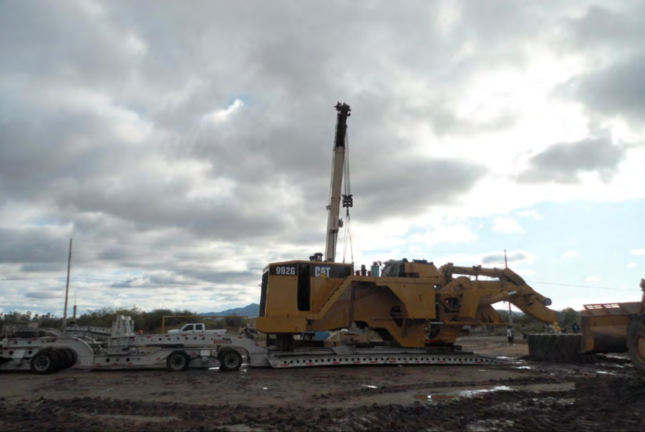
Assembly of front-end loader.
