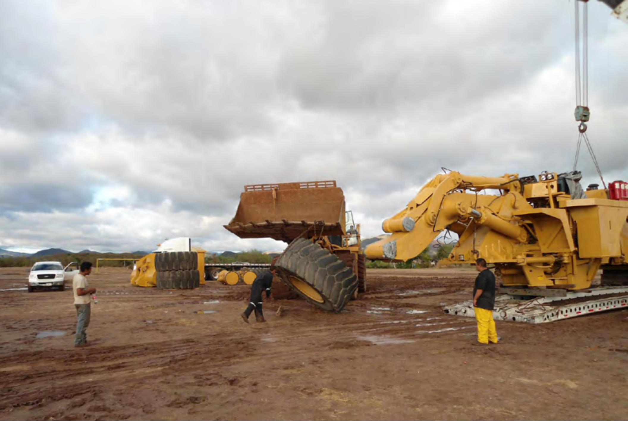
Assembly of front-end loader.
