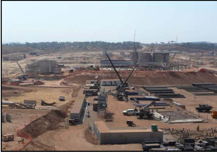
Tank Farm Area
