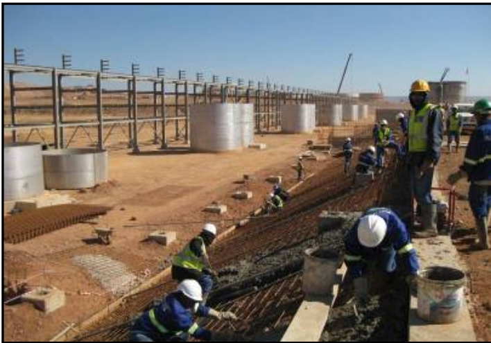
Electrolyte Pipe Rack
