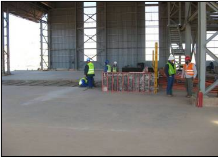
Heavy Truck Shop
