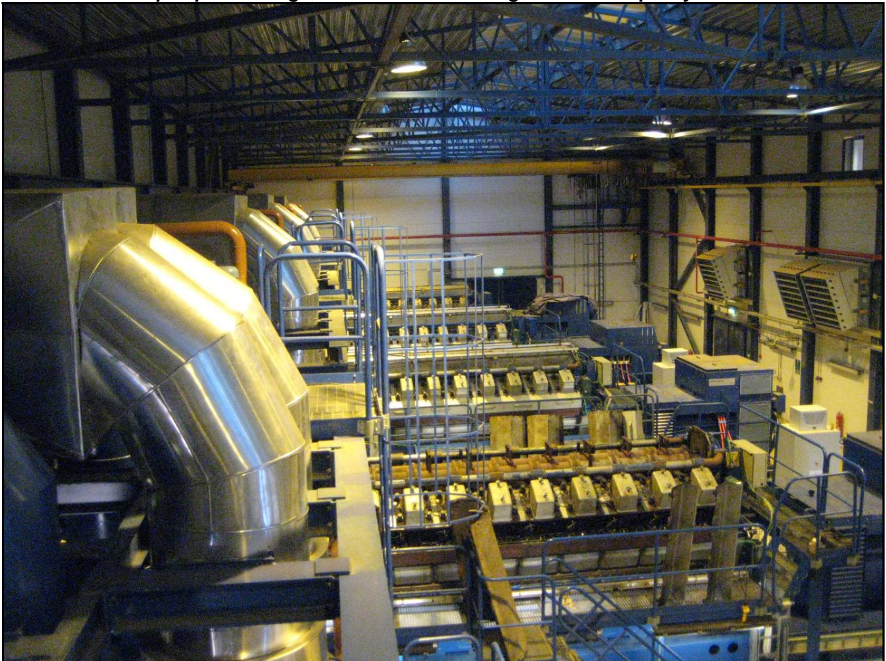
Power Station - 30MW
