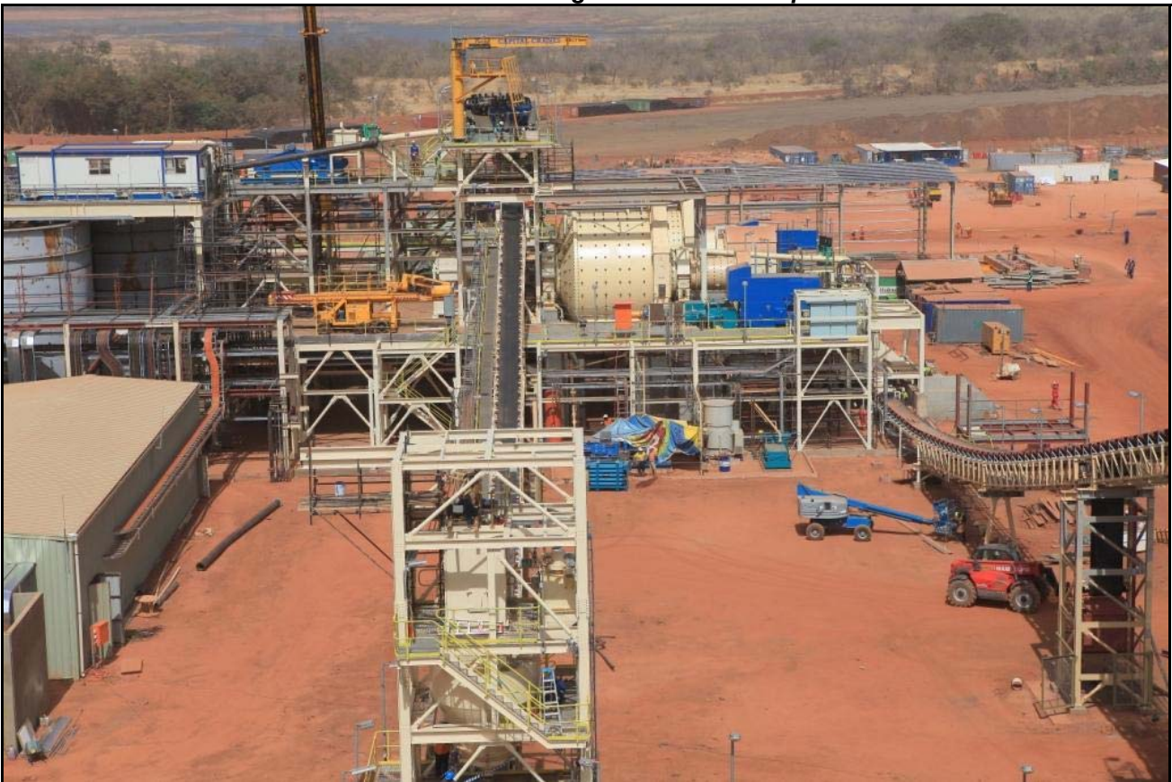
Treatment plant showing SAG and ball mills
