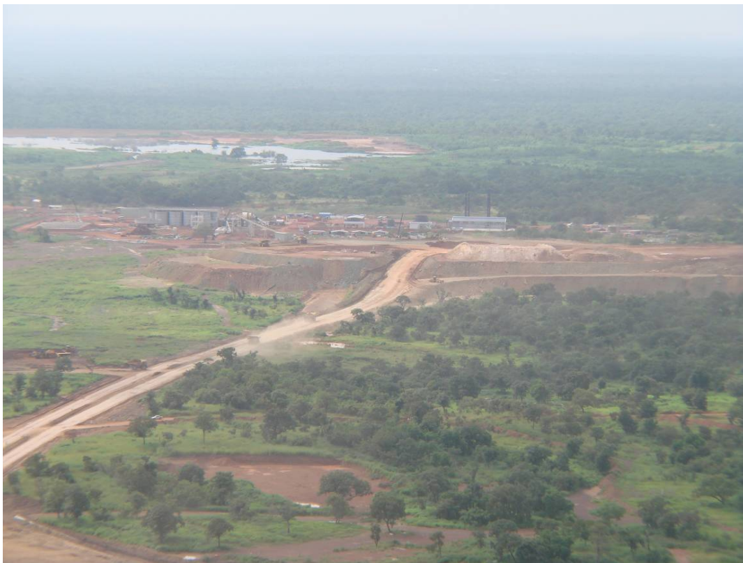
Trucks hauling construction waste and ore to the ROM pad with mill construction ongoing in background
