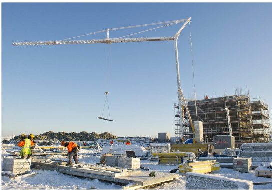
The foundation of the Tapuli primary crusher.
