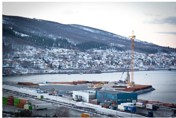
Construction is ongoing in the Fagernes Terminal in Narvik.
