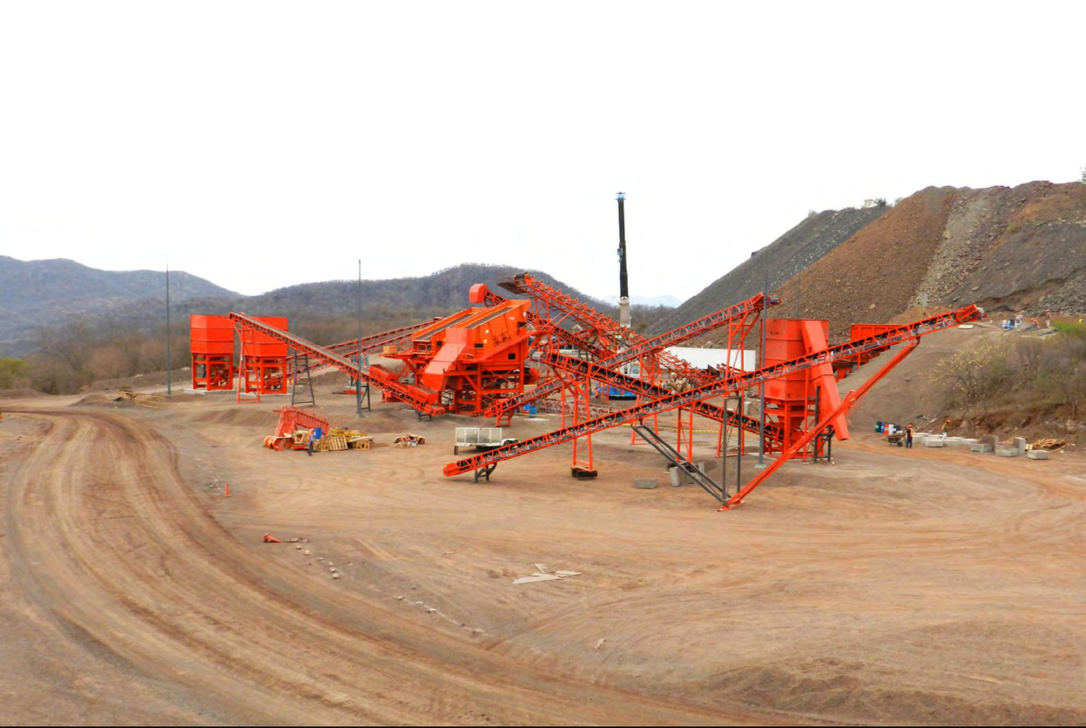
Final assembly of the crushers.
