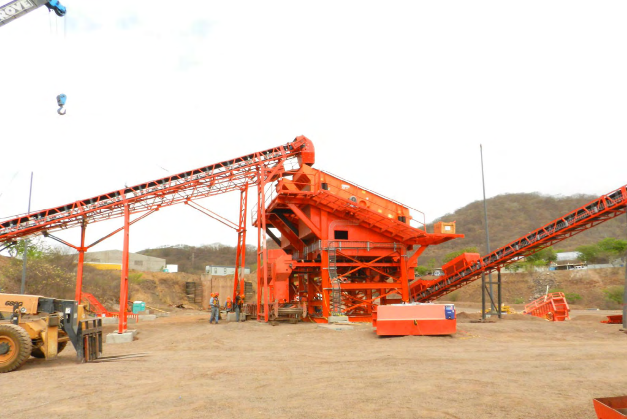
Final assembly of the crushers.
