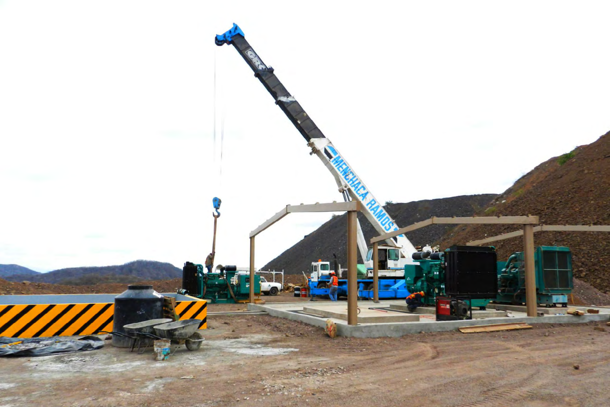
Installing generators for the crushers.
