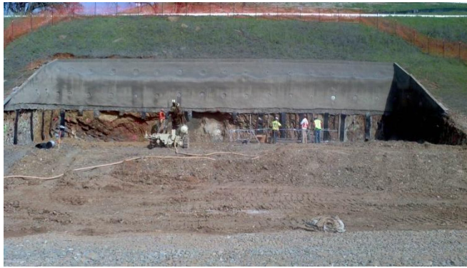
Photos of the first benches of excavation for the mill building showing ground support installation.
