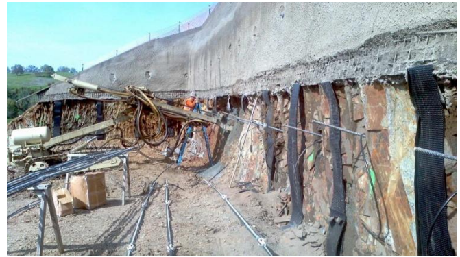
Photos of the first benches of excavation for the mill building showing ground support installation.
