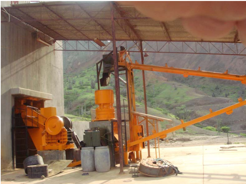
Crushing circuit with a 90% overhaul
