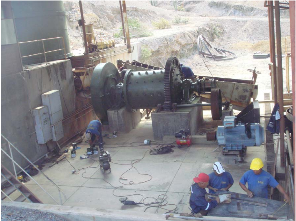
Mechanical work on the ball mill
