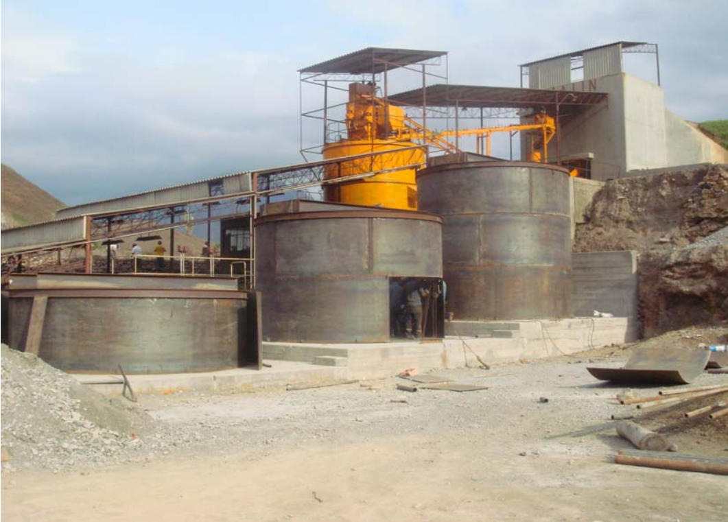
Lateral view of the new leaching tanks
