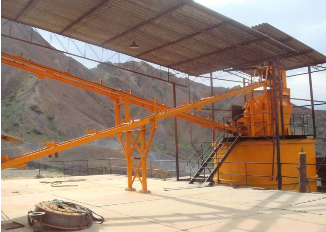
Crushing circuit with fines Bin after overhaul
