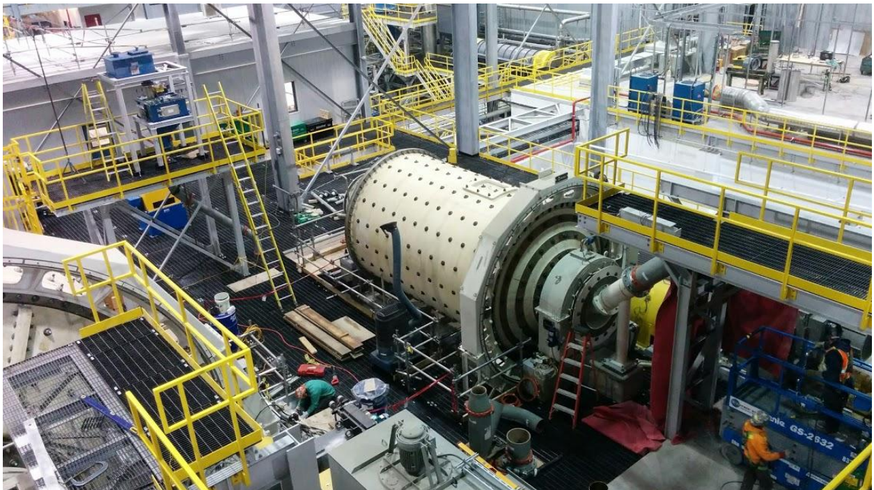
SAG and ball mill installation
