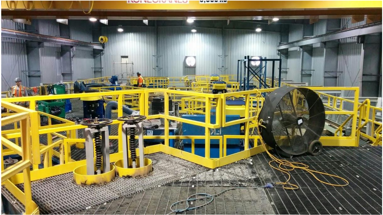
Top of the carbon-in-leach tanks with platforms installed
