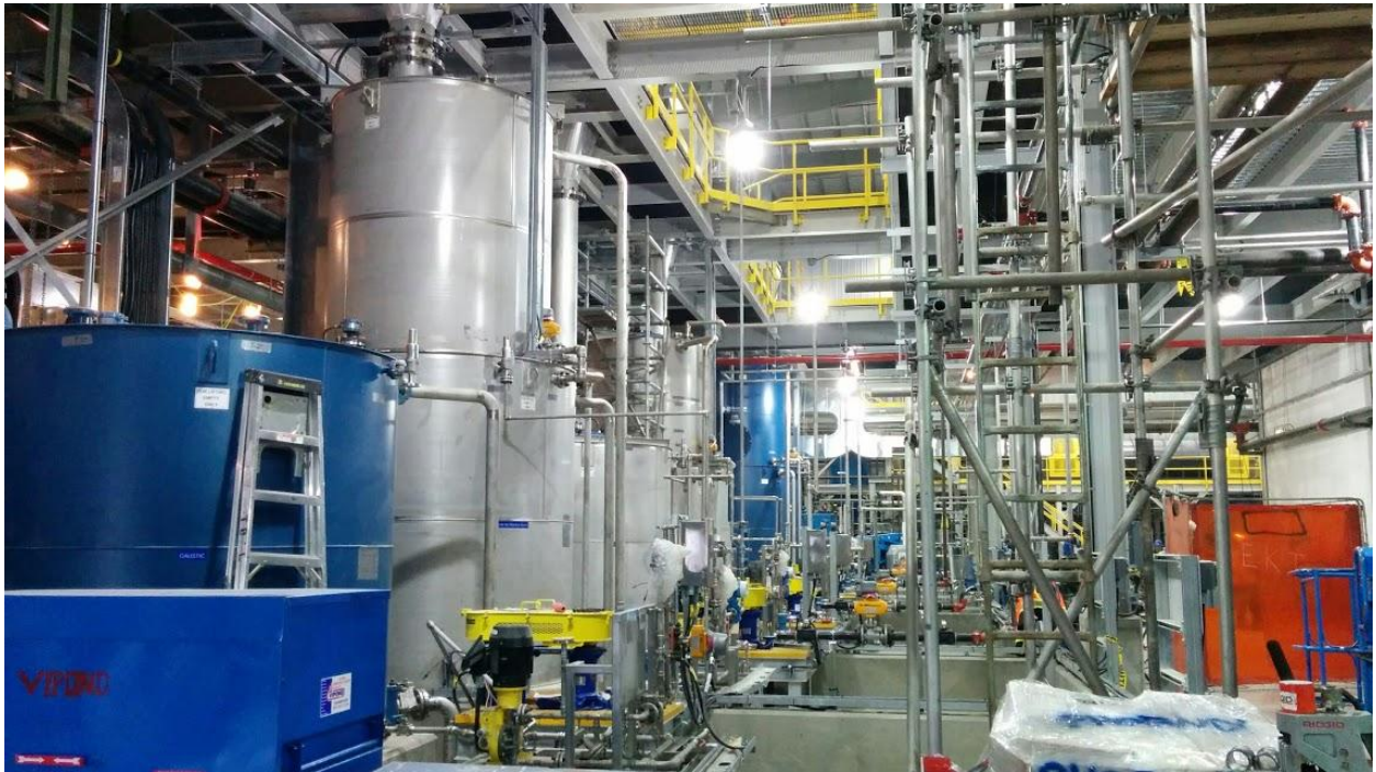
Reagents area commissioning
