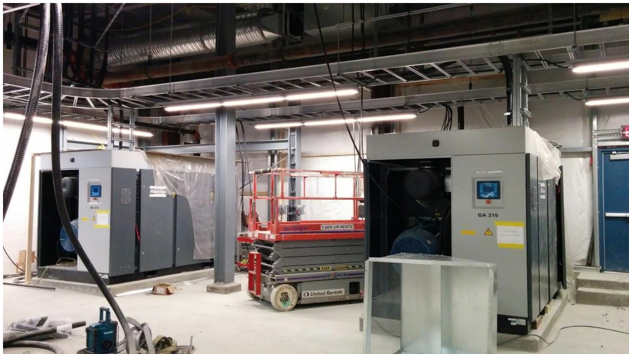
Compressor building installation
