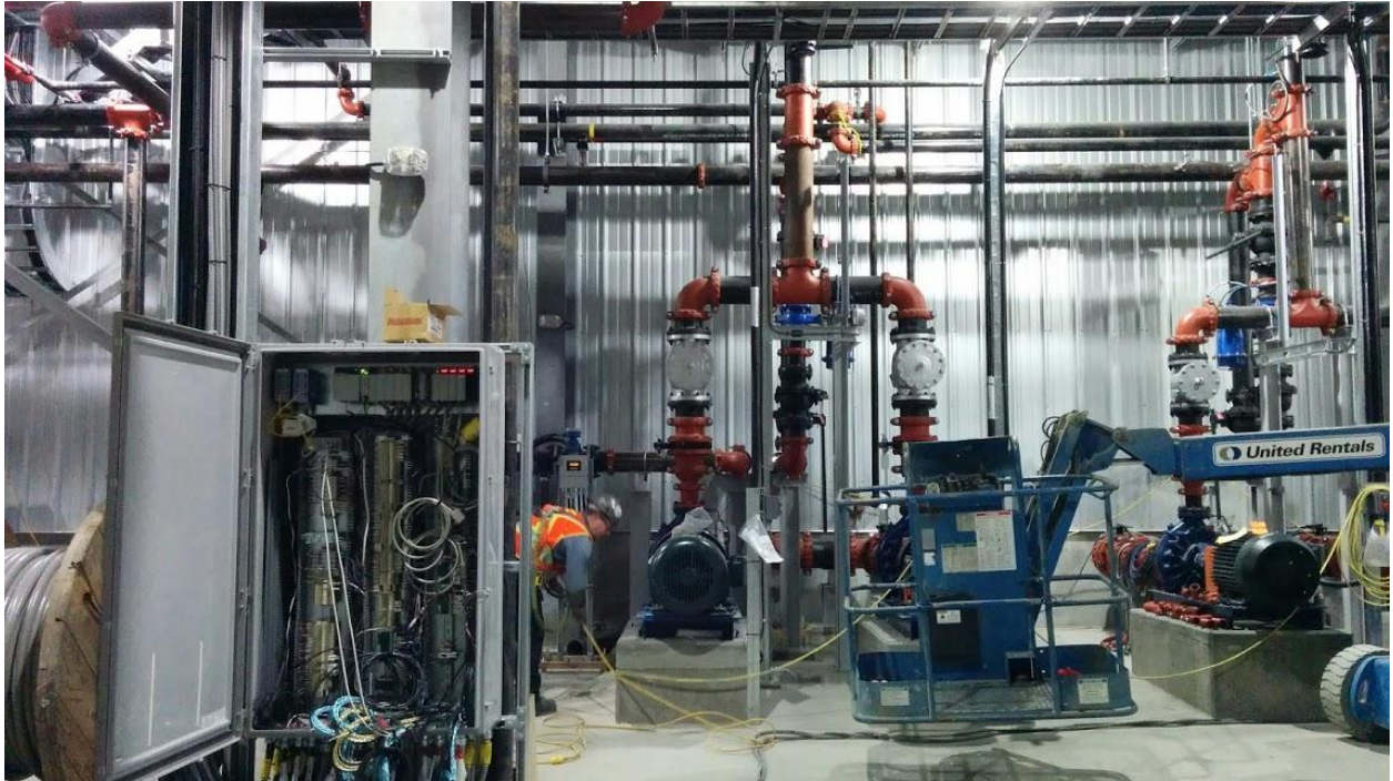
Installation of pumps in the grinding area
