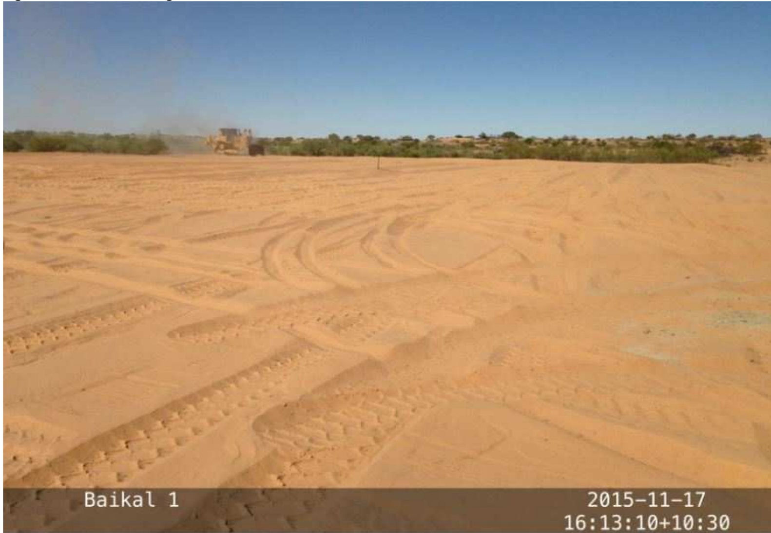
Figure 4: Baikal 1 Pad Being Cleared at PEL 444
