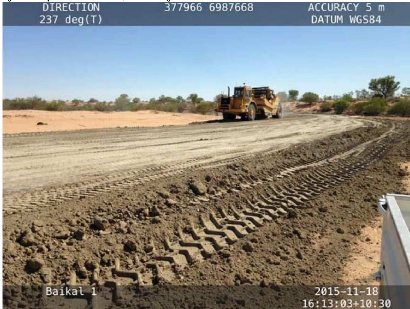
Figure 3: Drill pad under construction, Baikal 1 Target at PEL 444
