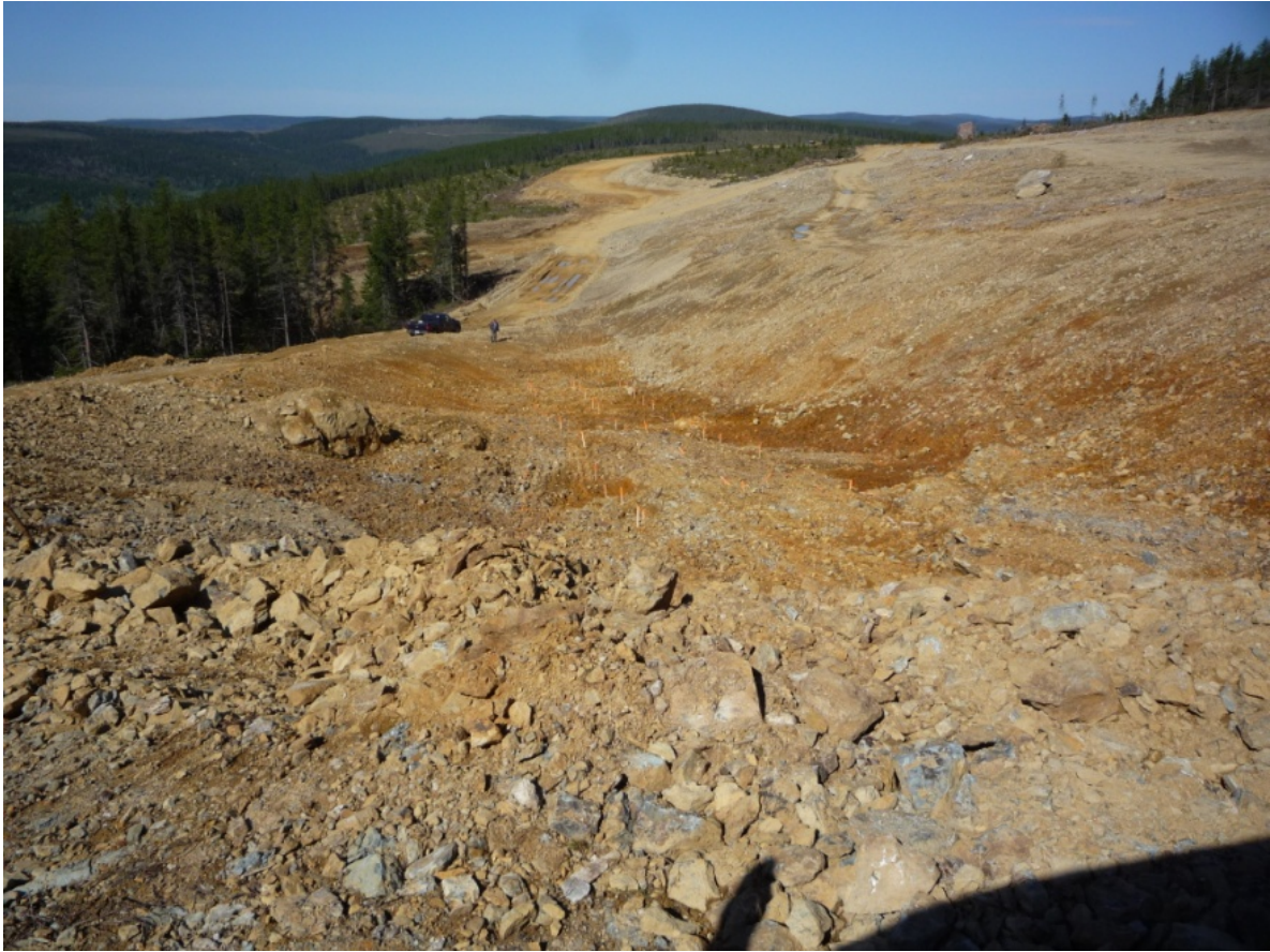
Figure 1: Access road and site preparation – Halfmile Project.
