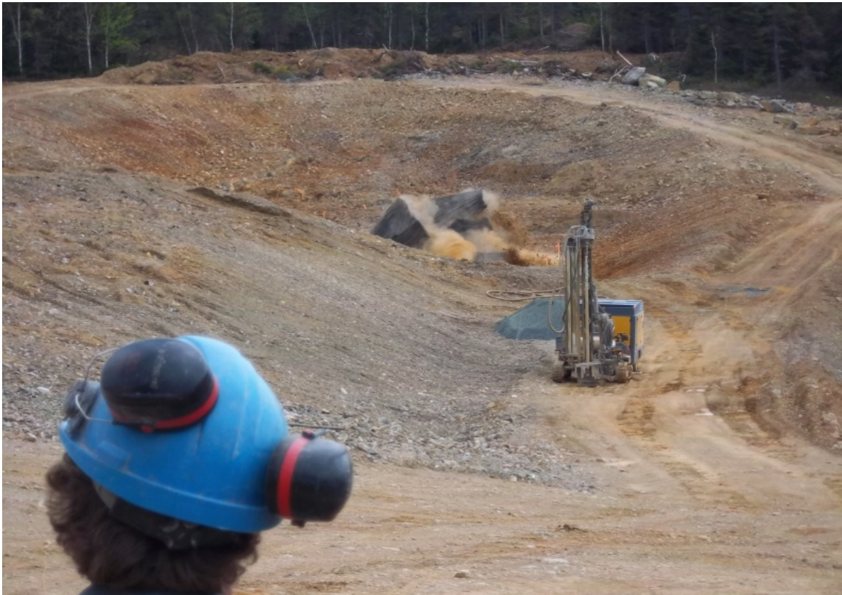
Figure 2: First blast of Halfmile access ramp.
