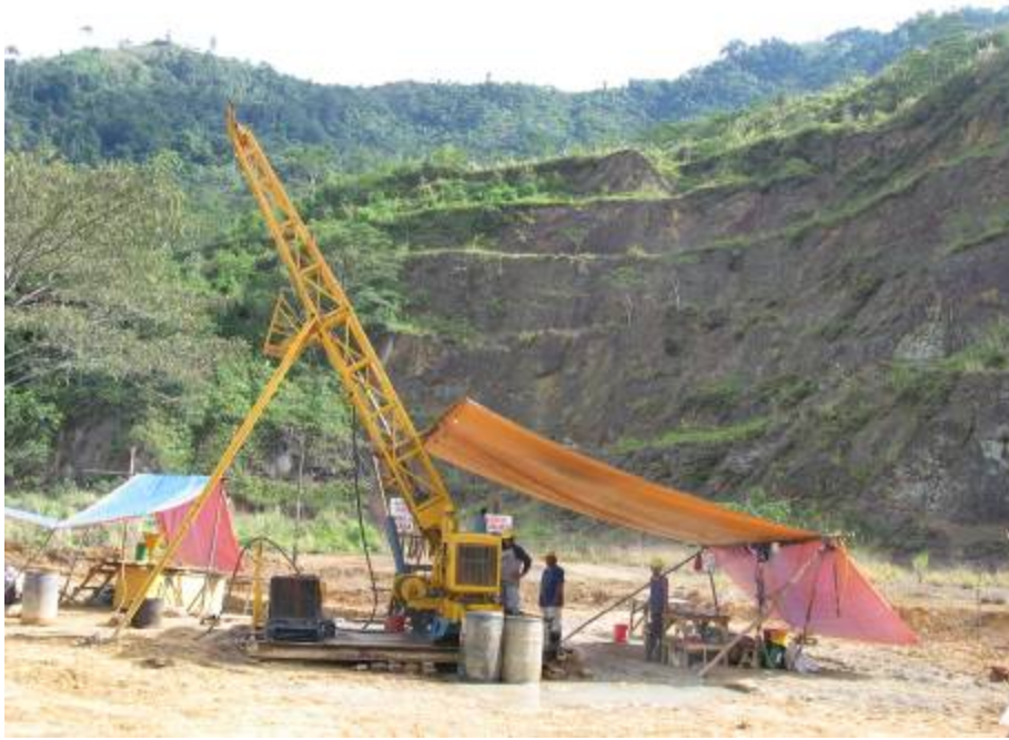
Above: Drilling TDG 16 at Tagpura Open Cut.
