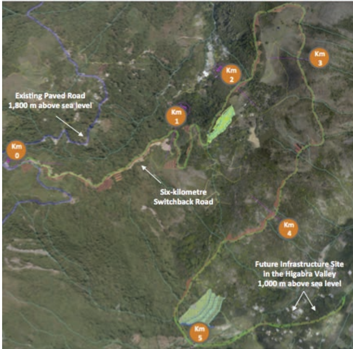
Figure 4: Six-kilometre Switchback Road Connecting Existing Main Paved Road with Future Infrastructure Site in the Higabra Valley
