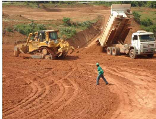
4 – Preparation of engineered fill;
