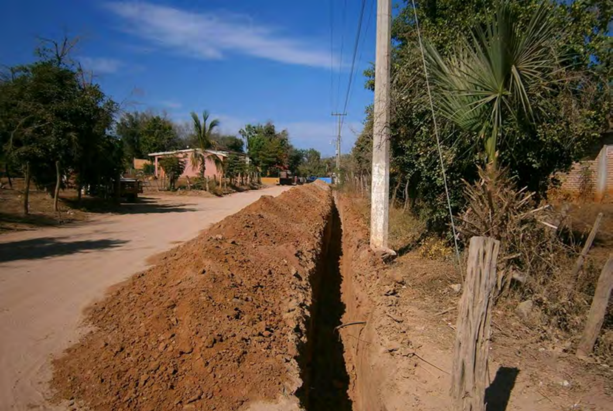
Preparation for haul road upgrading begins between the Palmarito and El Gallo deposit.
