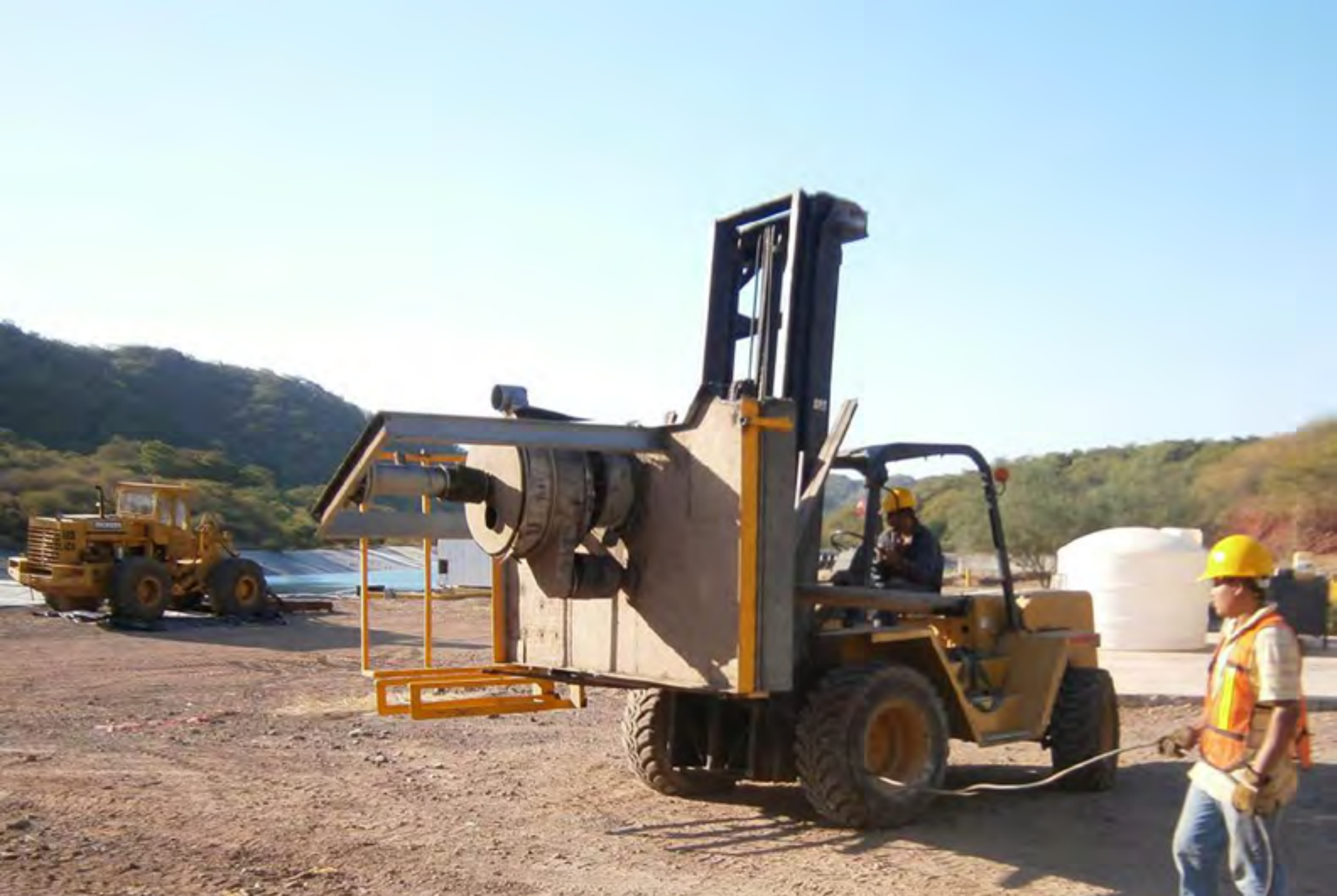
Dismantling of the old gold recovery plant equipment, now complete.
