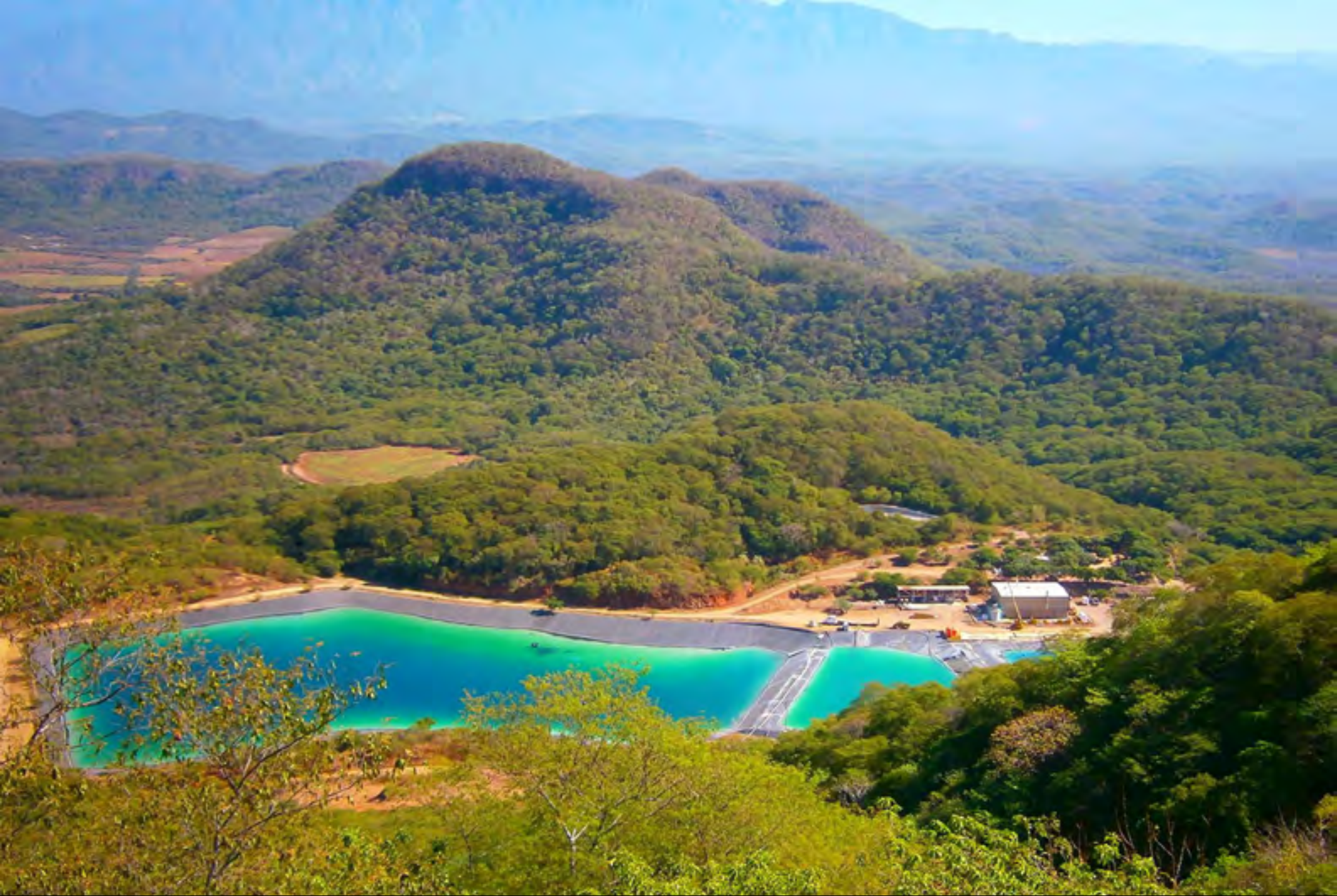
Looking down on the gold recovery plant and process ponds.
