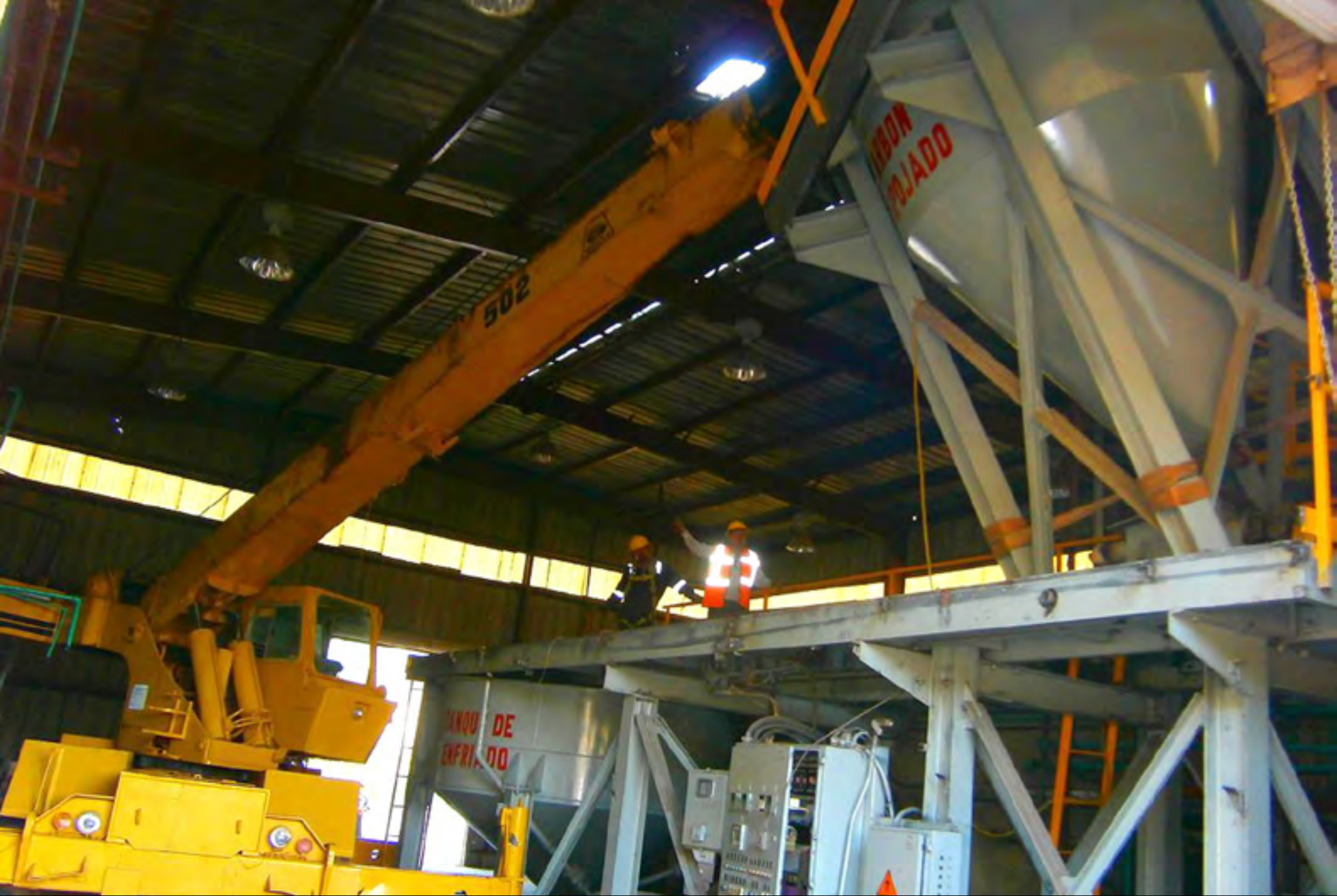
Looking inside the gold recovery plant building. The crane is in the process of removing older equipment that will not be used during mining.
