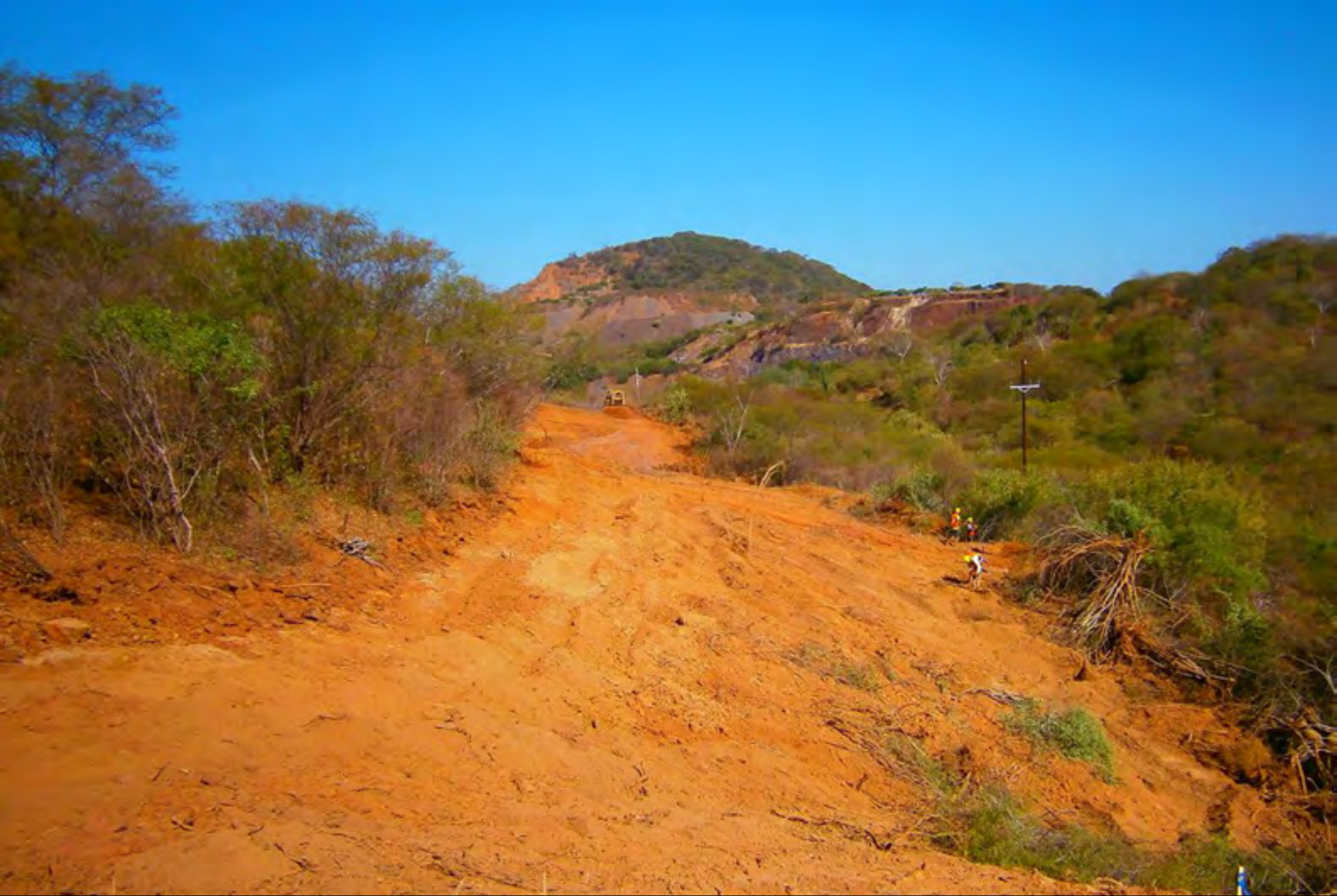
Clearing the way for haul road construction to the Lupita and Sagrado Corazon deposits. Looking north towards the previously mined area.
