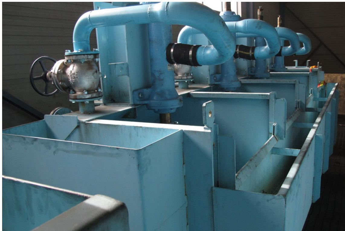
Photo 2: Assembly of floatation cells in situ at the Woxna Plant
