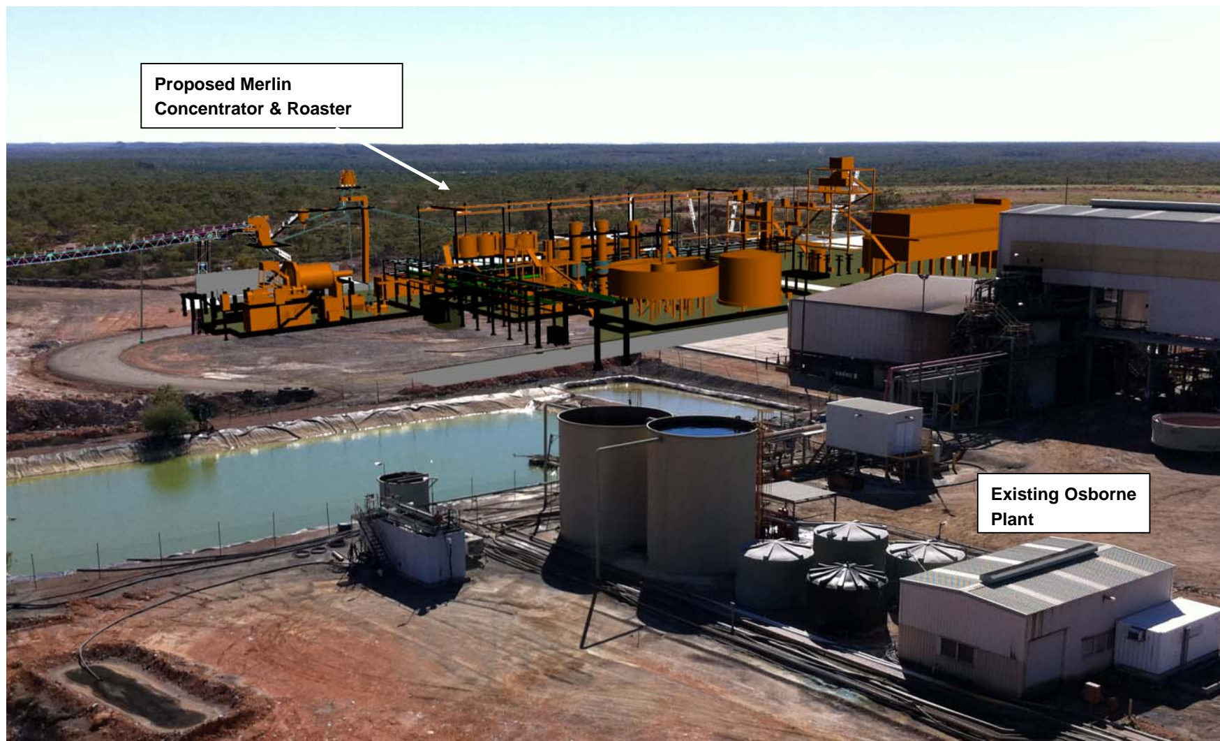
Figure 8. Proposed Molybdenum/Rhenium Processing Plant, adjacent to existing Osborne plant
