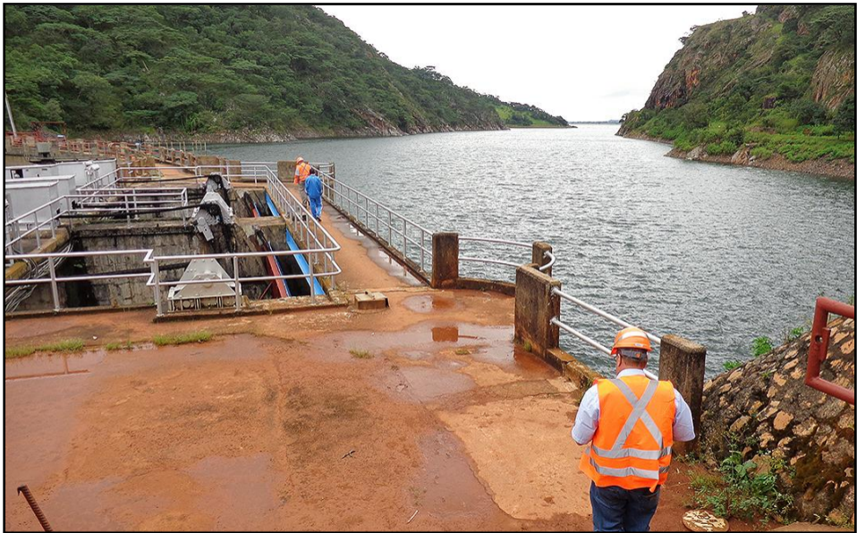
Nzilo 1 hydroelectric power plant, Katanga, DRC
