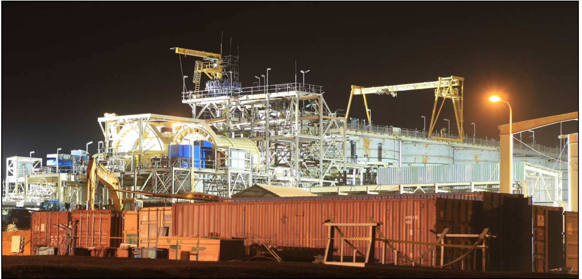
Plant showing SAG and ball mills in yellow and CIL tanks in background
