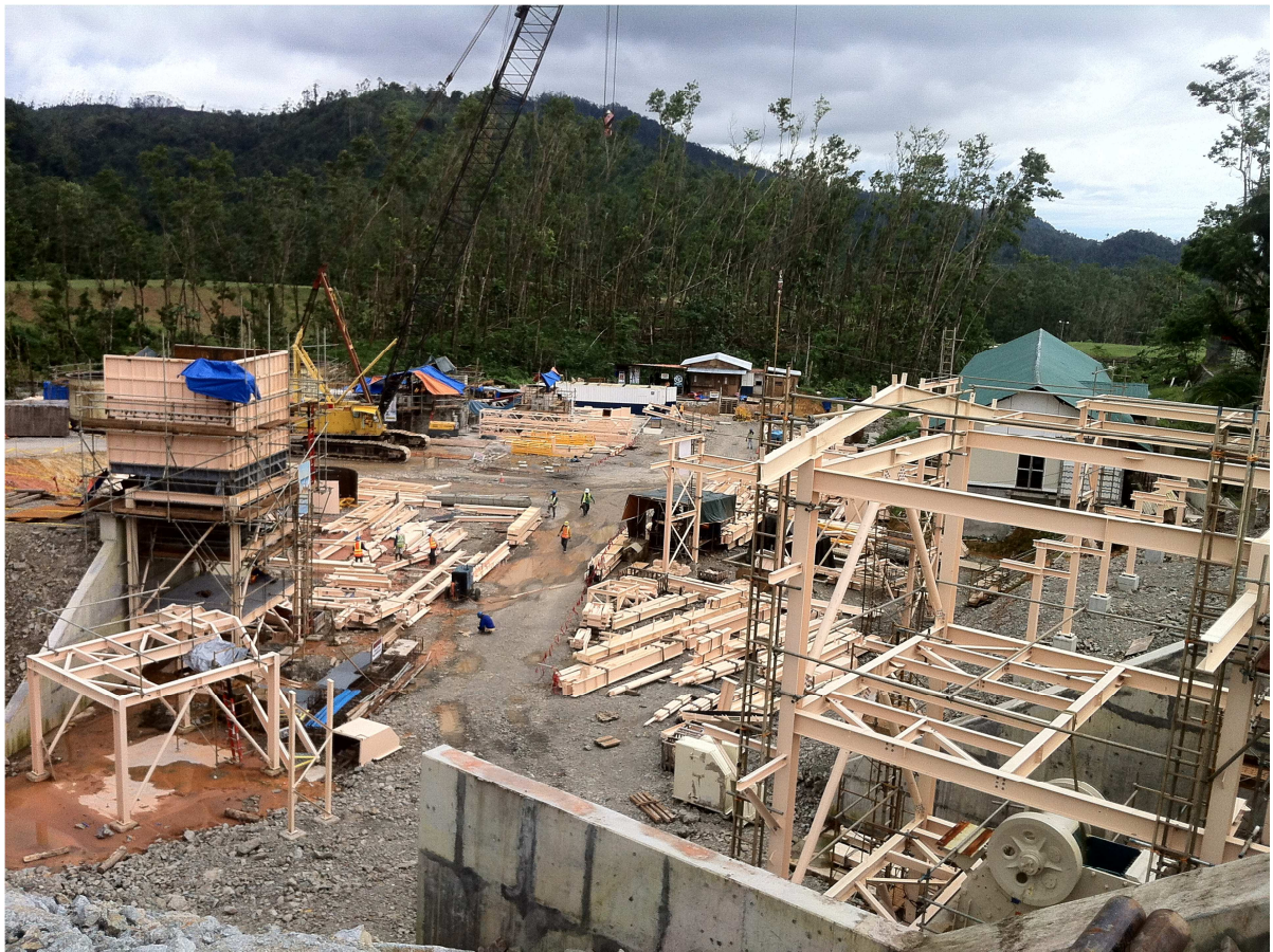
Photo 2. Installed crusher on the right and emergency feed station on the left. The SAG mill foundations are behind the 150 tonne crane which will be used to lift the SAG mill components onto the concrete foundations.
