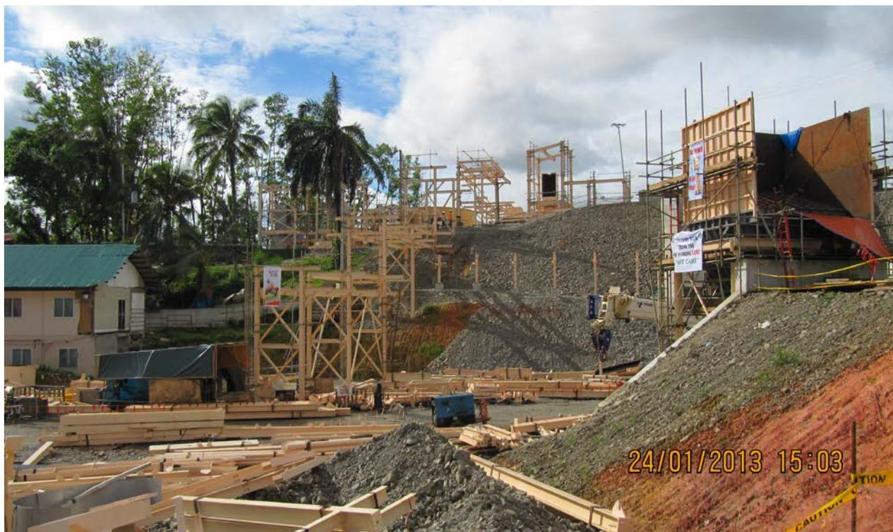
Photo 3. Pipe rack construction from SAG mill to leaching circuit on the left with the emergency feed station on the right.
