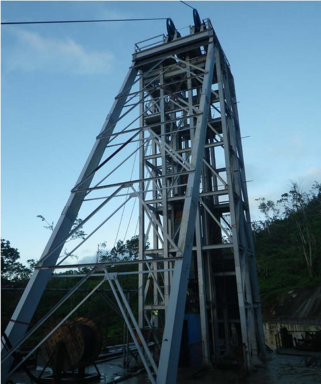
Photo 1. Completed Saga Shaft headframe
