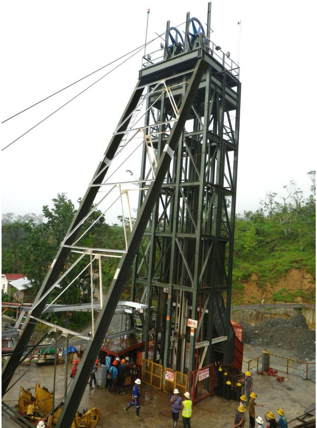
Photo 1: Completed Saga Shaft headframe
