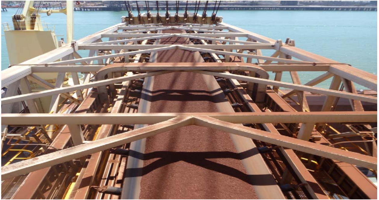
Spinifex Ridge Iron Ore being conveyed to the Utah Point shiploader.
