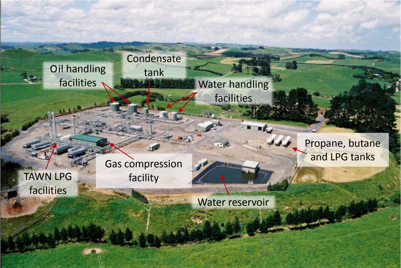
Figure 2 – Waihapa Production Station
