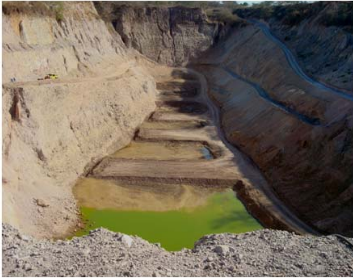
Taurus pit after being dewatered
