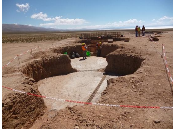
Foundations for Lime Plant Silos
