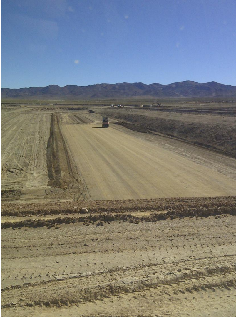
Evaporation pond under construction
