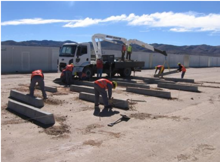
Foundation construction for camp containers
