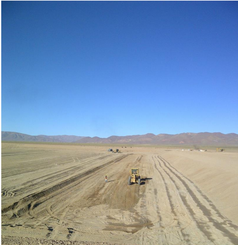
Evaporation pond under construction
