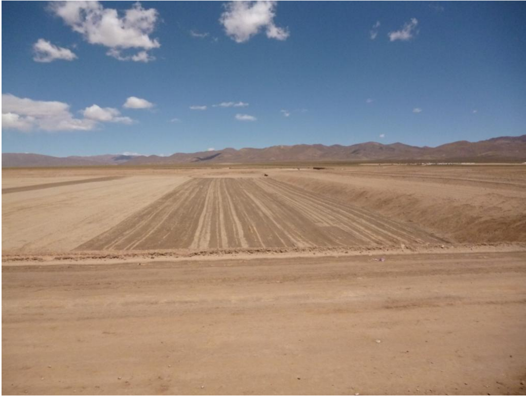
Evaporation pond under construction
