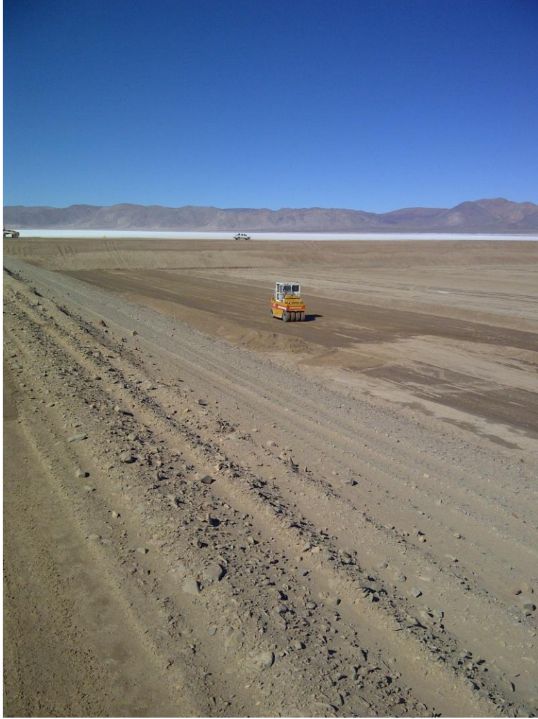
Evaporation pond under construction
