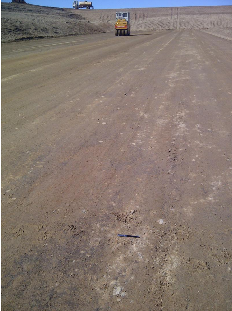
Evaporation pond under construction
