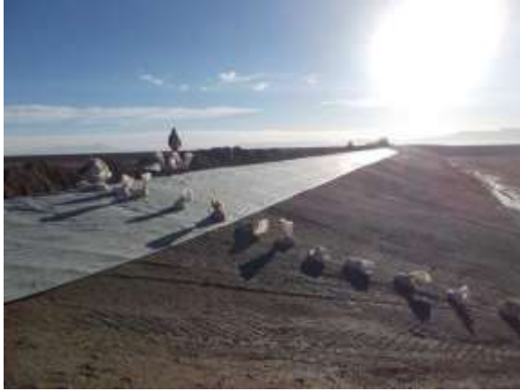
Evaporation Pond Lining
