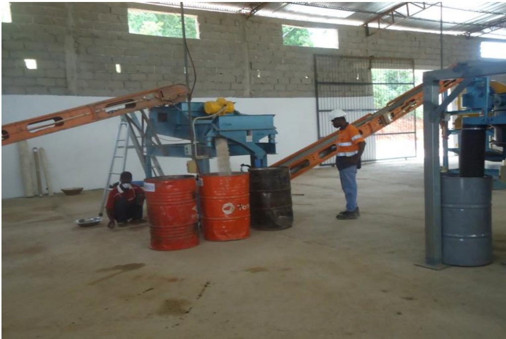
Figure 5 – Secondary Plant in operation
