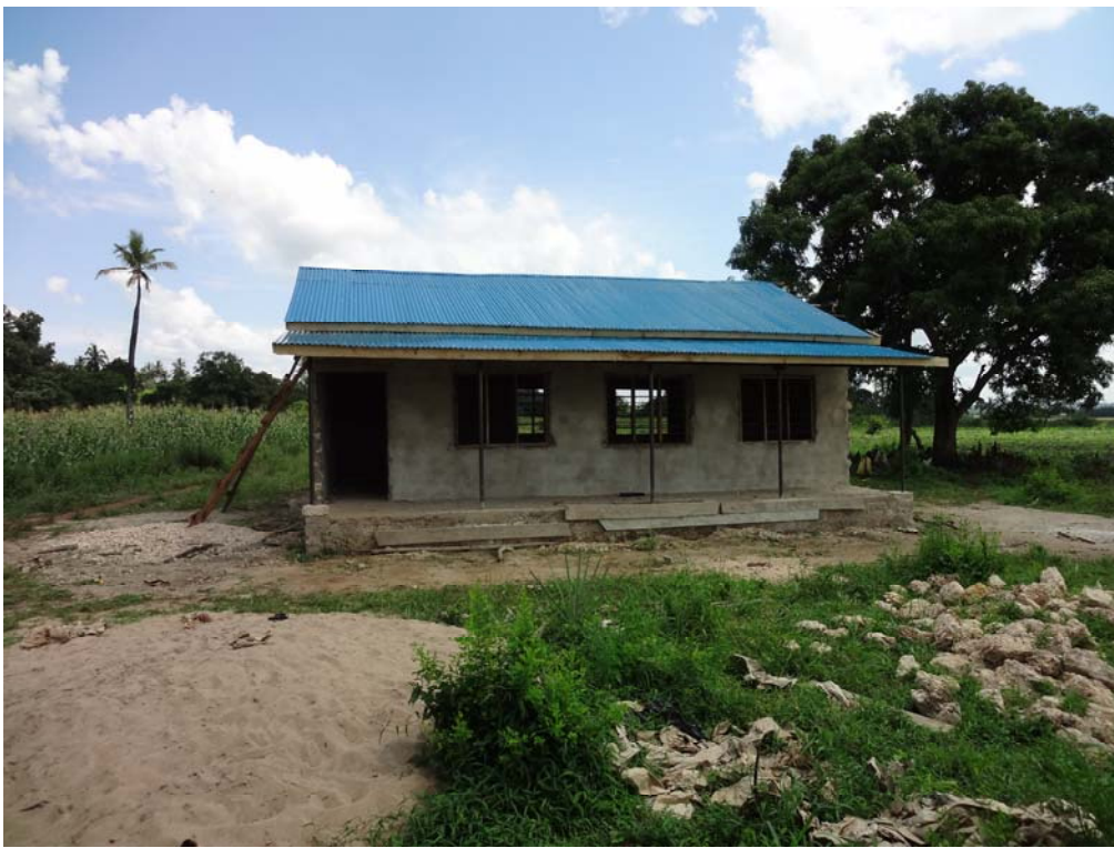
Classroom at Bumbuni nears final completion
