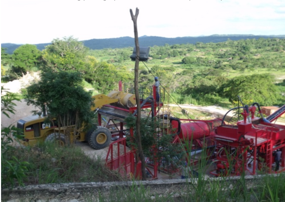
Cat 928 FEL feeding mined material into the Primary Plant
