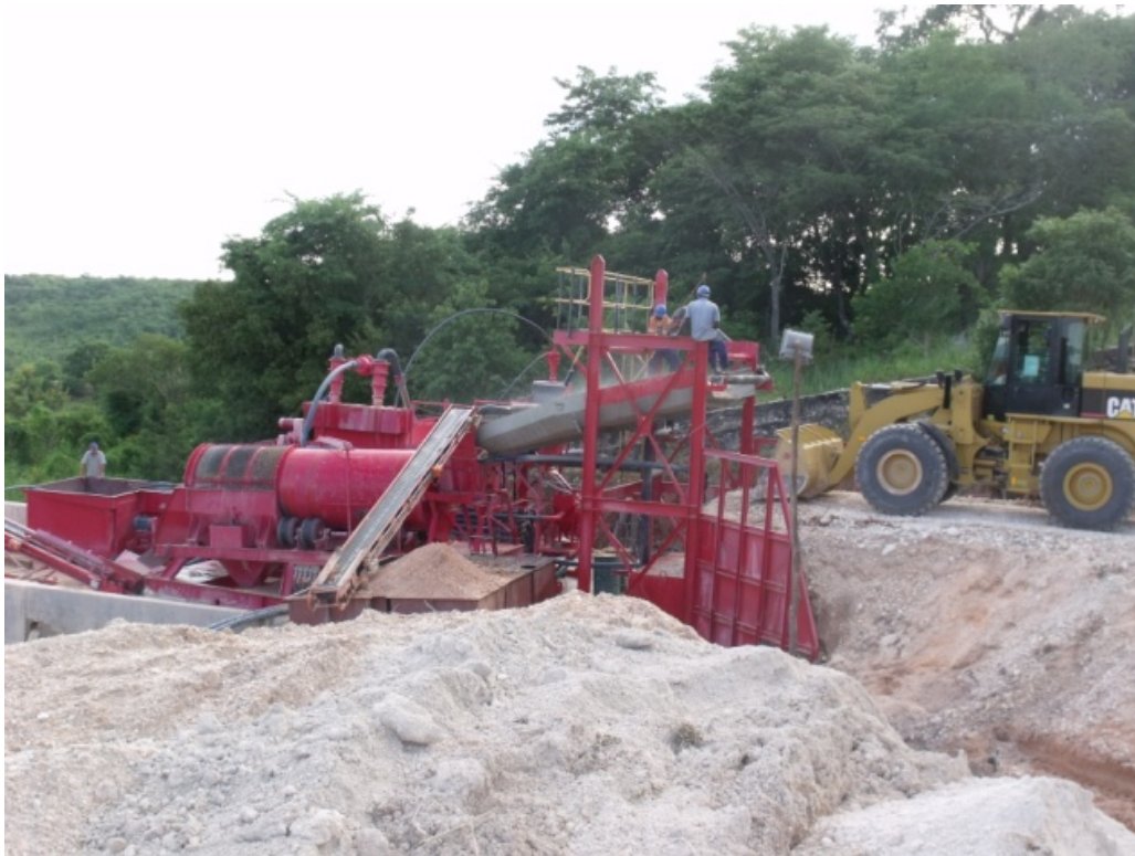
Primary plant in operation
