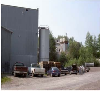
Ryan Lake mill building
