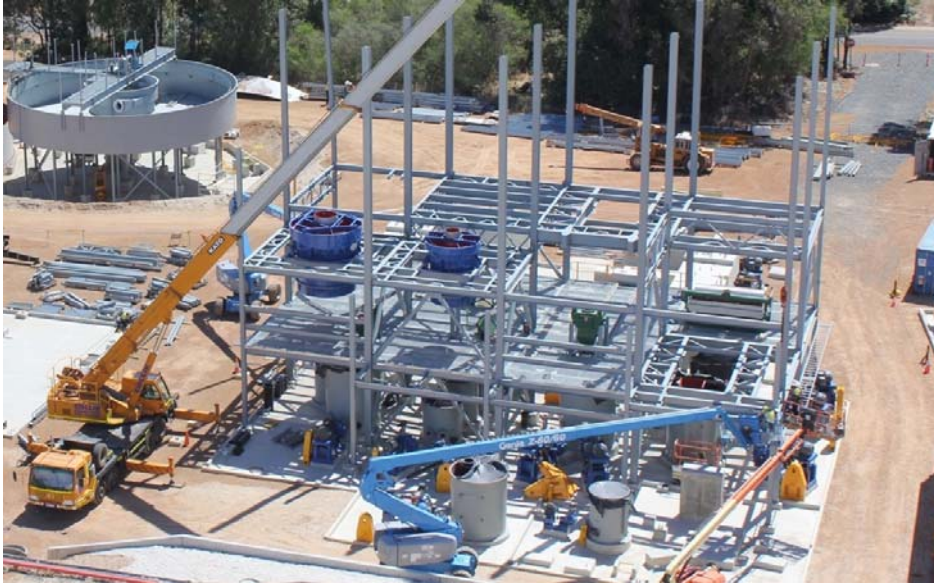
Work on the new chemical-grade plant as part of the Stage 2 Expansion at the Greenbushes Lithium Operations.
