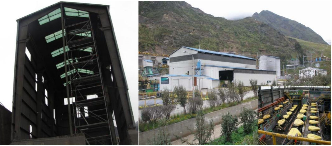
Figure 2: Left: Refurbished Crushing-House – Santander Project. Right: 2,000-tonne-per-day processing plant presently being installed and re-commissioned at Santander (inset: flotation cells).
