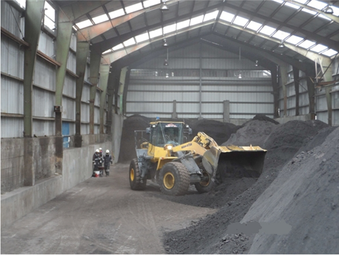
Figure 1: Zinc concentrate shed at Trevali's Santander Mine
