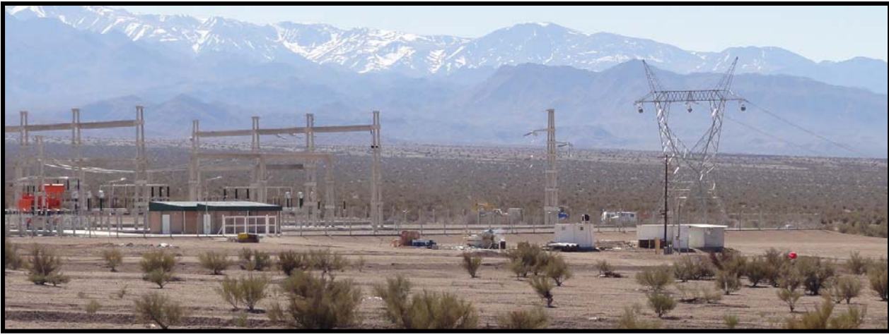
Photo 1: New 500kVA power line connecting to the new Calingasta substation. The Casposo Mine will move from diesel to grid power in the month of December
