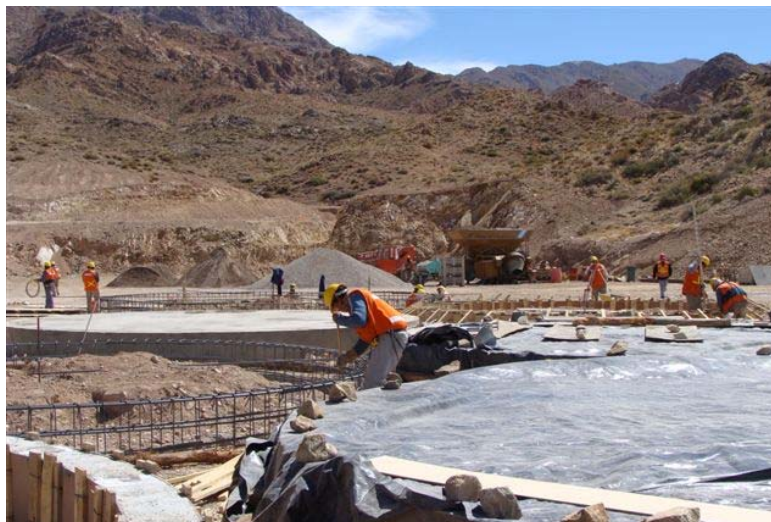
Leach tank concrete rings under construction
