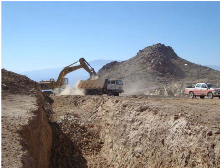
Excavation for ore stockpile withdrawal tunnel
