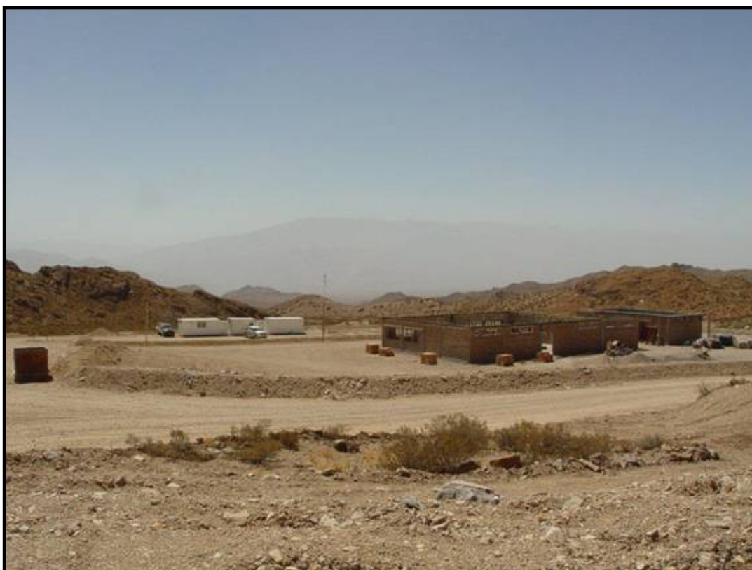
Photo 4 - Canteen and First Aid and Safety buildings under construction.
