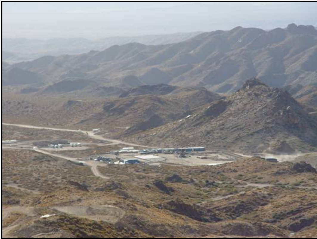
Photo 1 - View looking SE from Kamila deposit to plant construction site.
