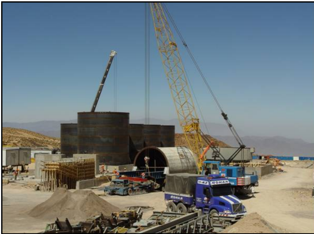
Photo 2 - Cobalt mill in the foreground of leach tanks.
