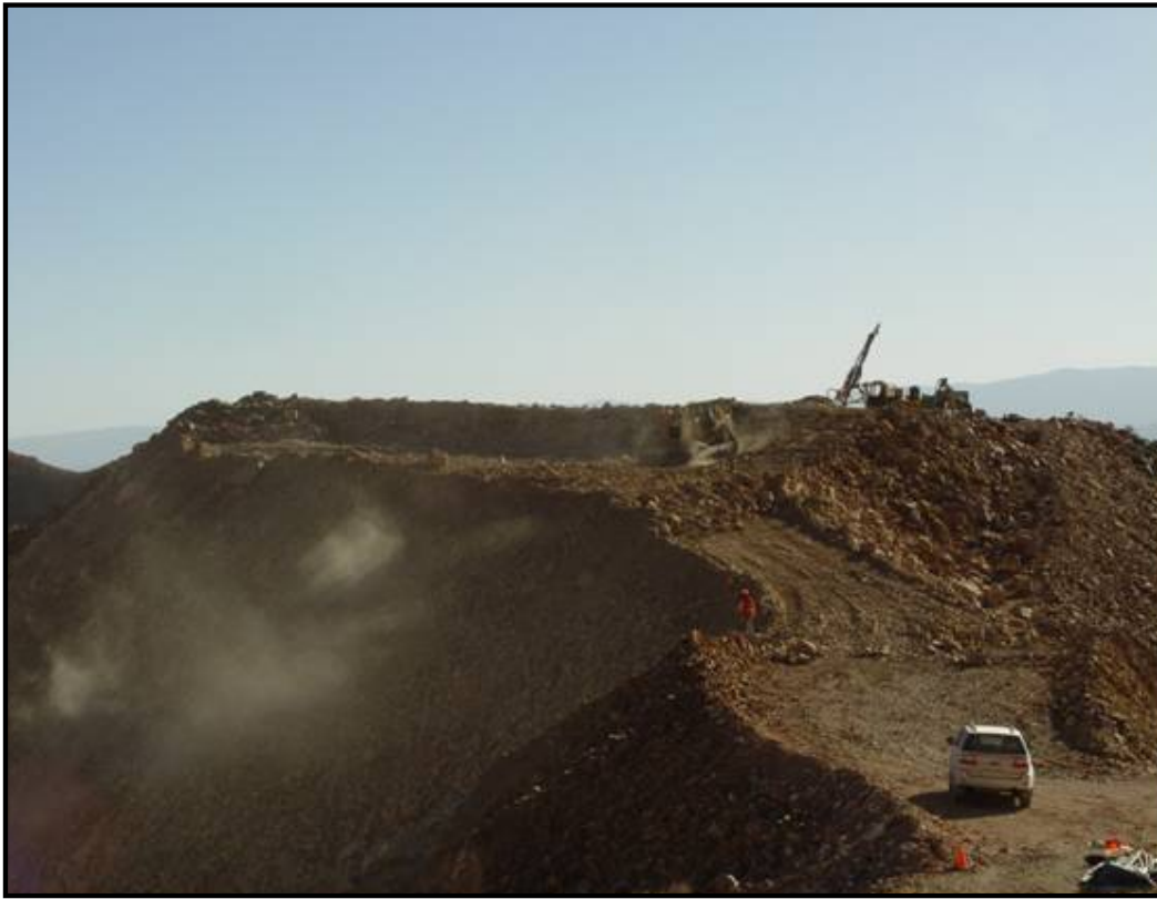
Photo 5 - Initial pre-strip and road construction to the Kamila open pit.
