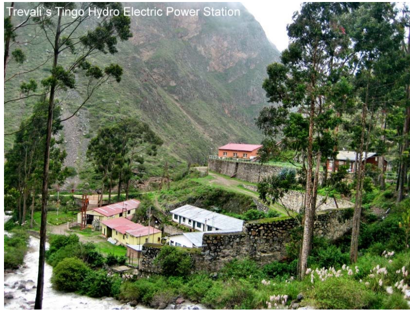
Figure 1. Trevalli's Tingo hydroelectric generating station
