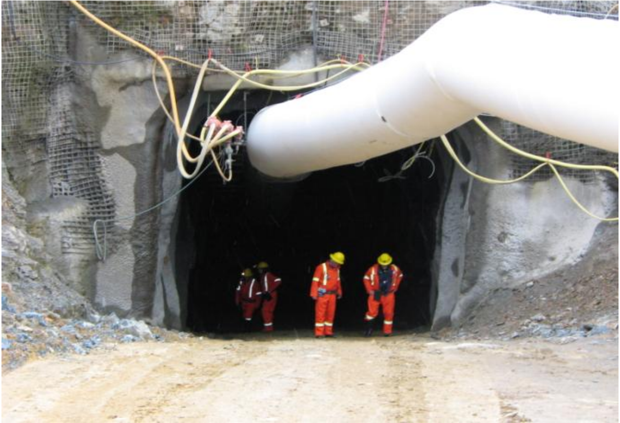
Figure 1: Mine Adit development at Trevali's Halfmile Deposit, New Brunswick
