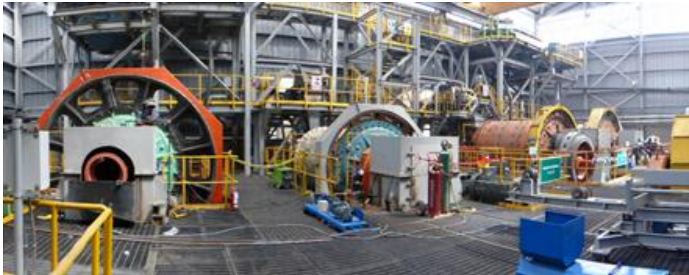
Figure 2. Grinding circuits at Santander mill.
