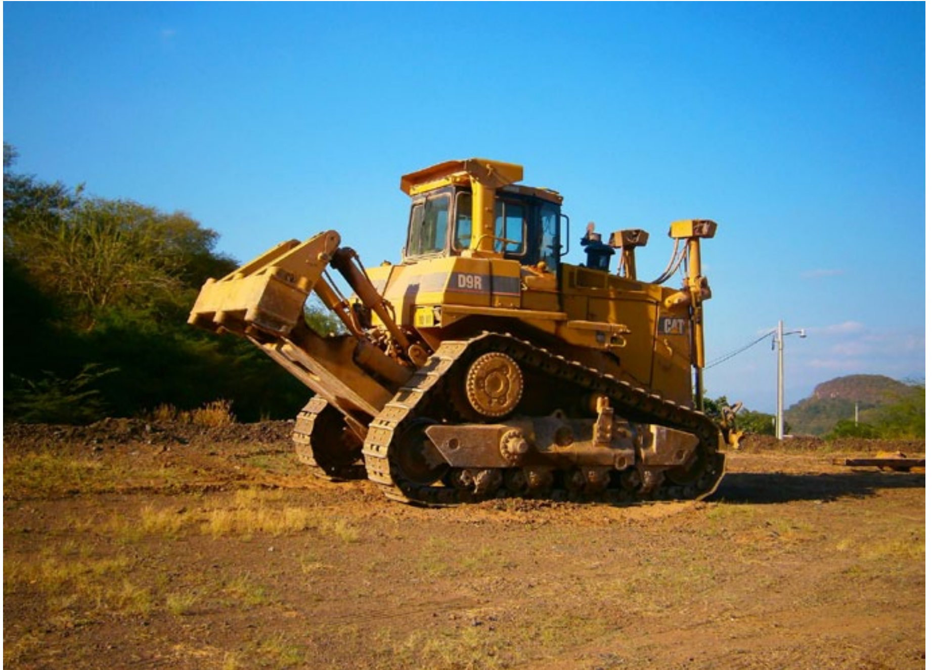
Caterpillar D9 Bulldozer being assembled to start haul road construction.
