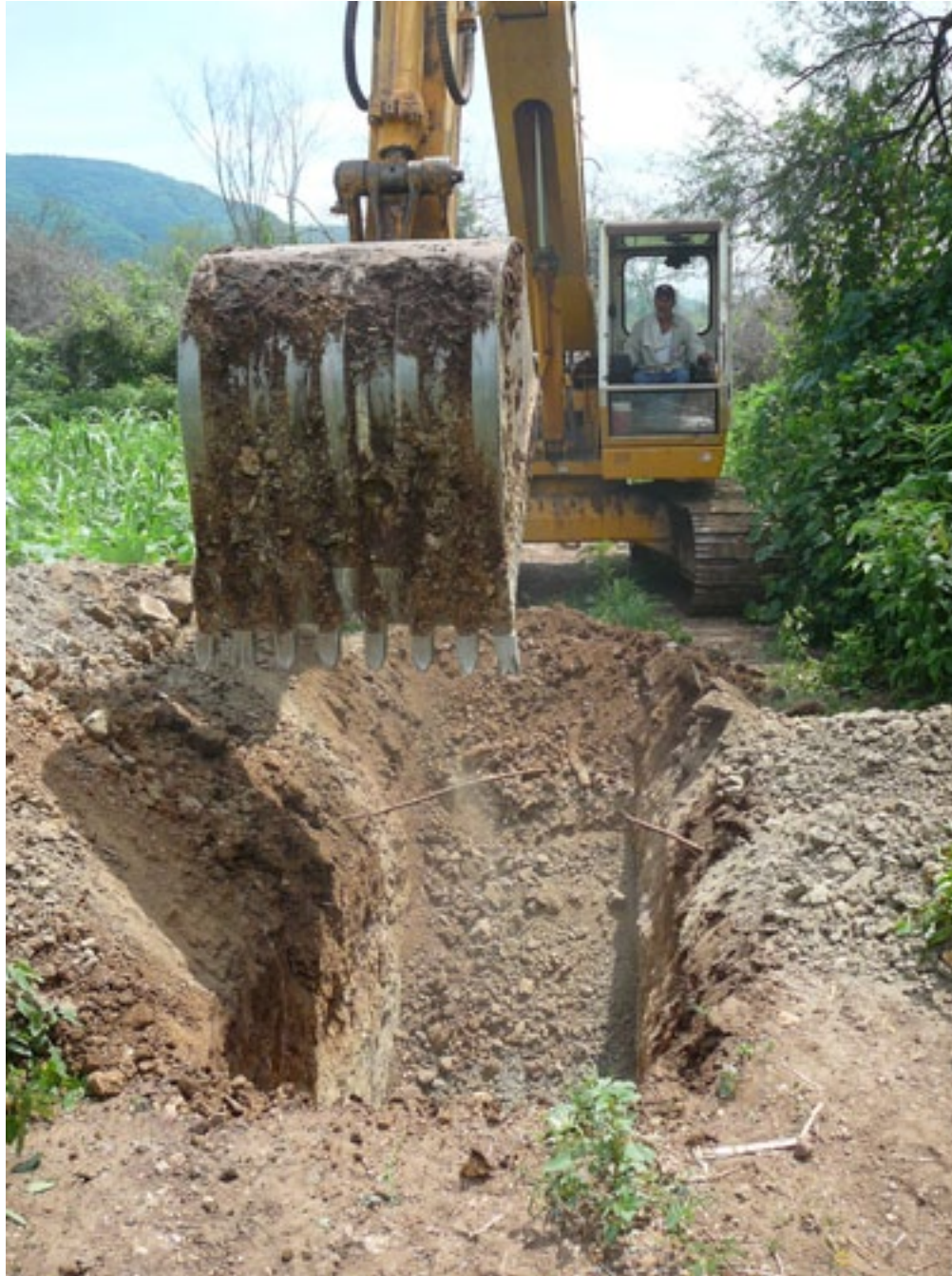
Tailings storage facility structural foundation investigation at El Gallo. Variable strength and permeability testing pending lab analysis.
