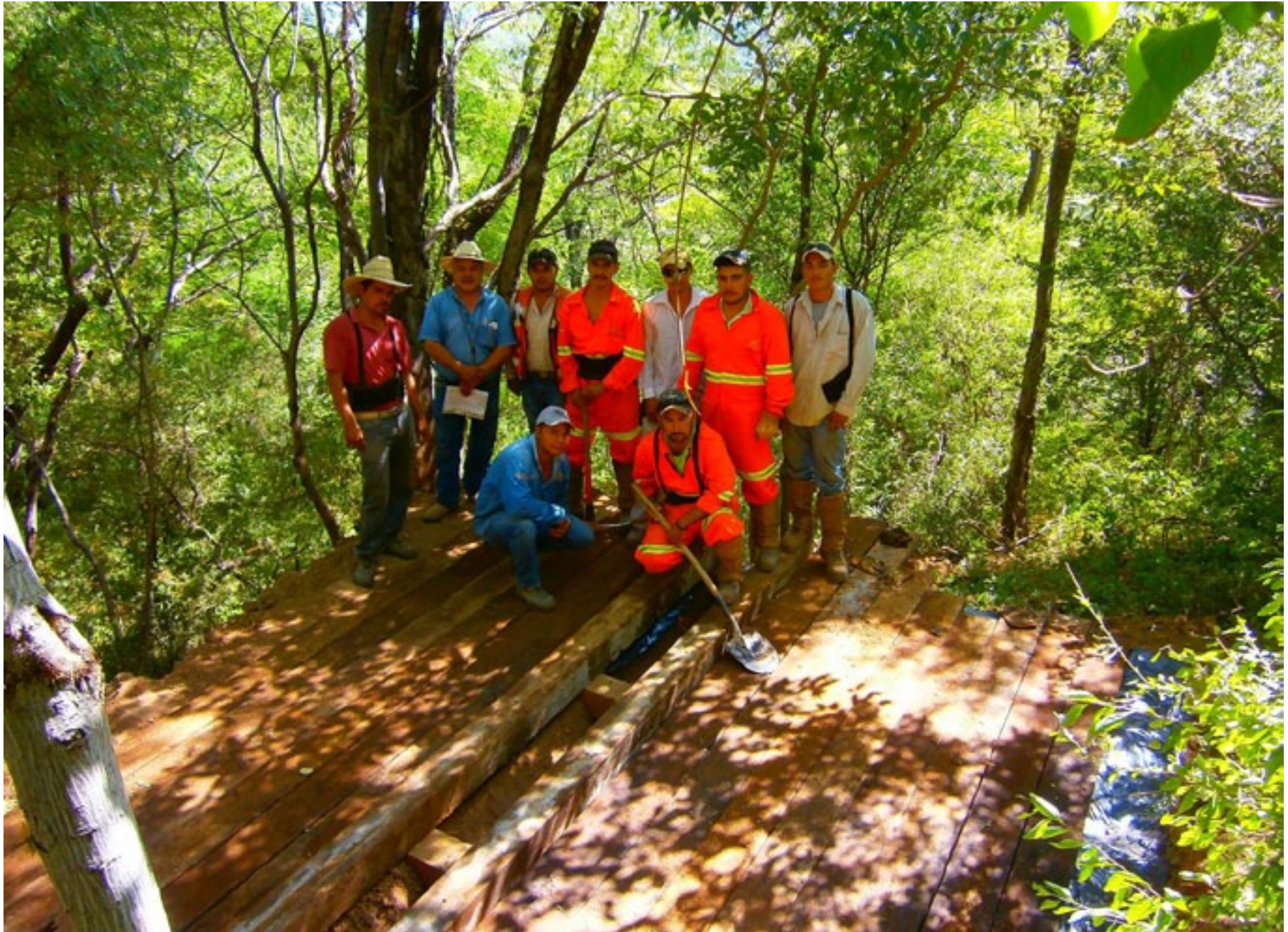
Mexico team: Building a platform to complete condemnation drilling at El Gallo, which are designed to minimize the environmental footprint and measure only 4 x 4 meters.
