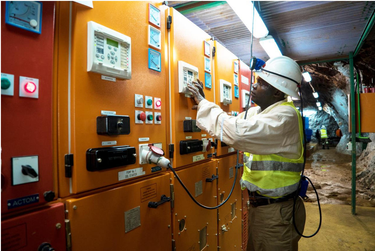
Figure 9: Pumping station, part of the underground infrastructure upgrading.
