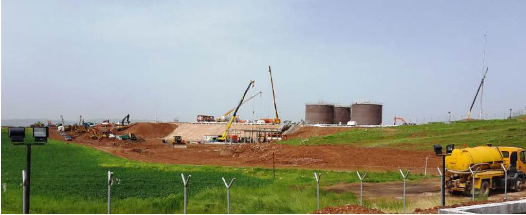
Shewashan EPF under construction – April 2017
