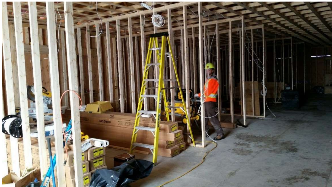
Electrical installation commenced
