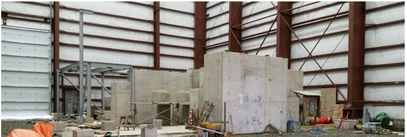
Steelwork around mill and Mill Plinths
