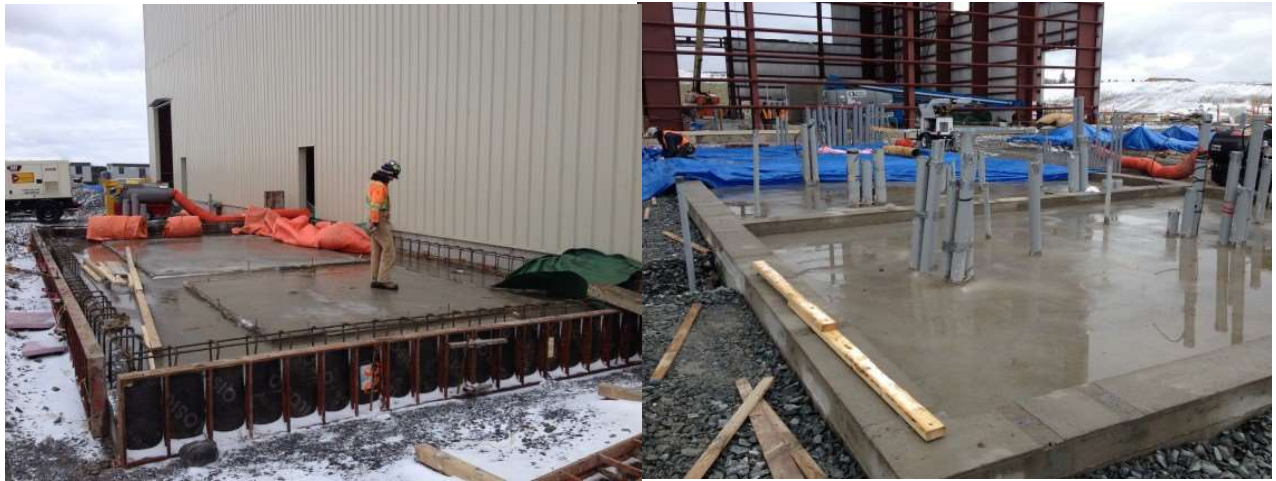
Lube Room Area MCC Foundation
