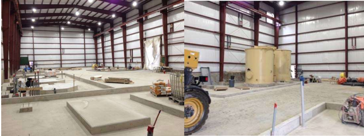
Reagent Building – Concrete Completion & Mechanical Installations
